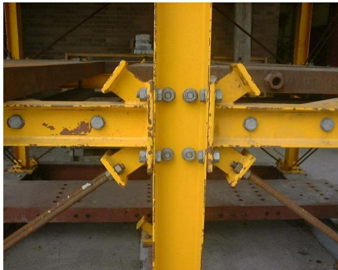
*Figure 4: Beam to column connection (Ventura et al., 2003)*
