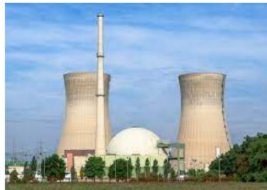
Figure 7: Nuclear power plant
