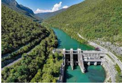
Figure 6: Run-of-river hydropower plant
