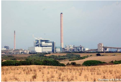
Figure 8: Natural gas power plant
