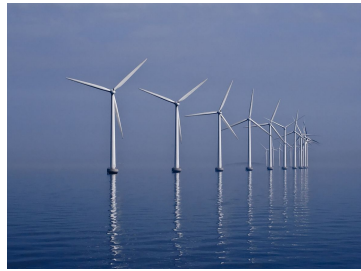
Figure 5: Wind offshore power plant
