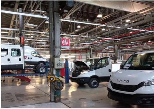
Figura 64: lampade a ioduri metallici in area Ovest
