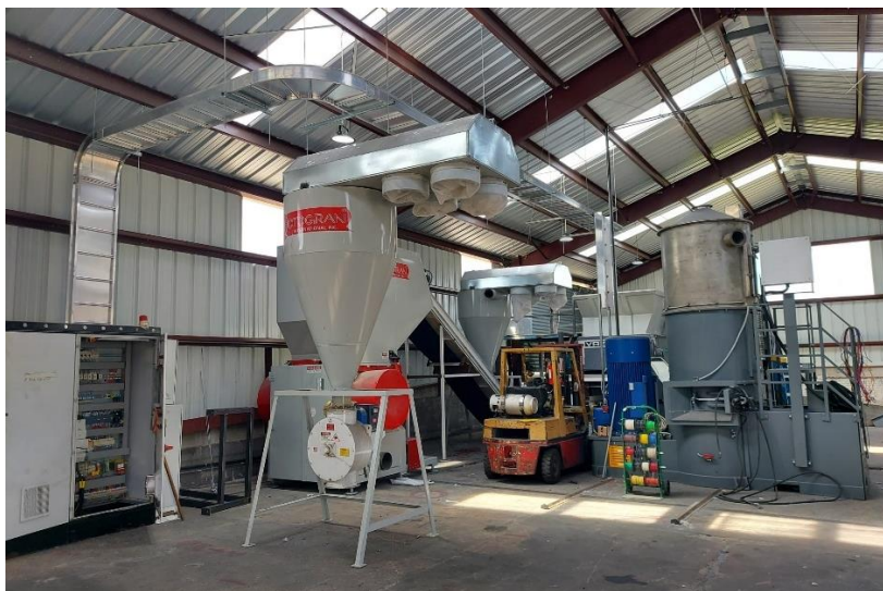
Figure 424 hybrid line under construction
