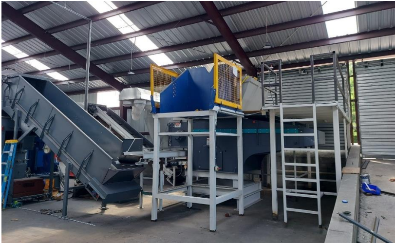
Figure 413 hybrid line under construction
