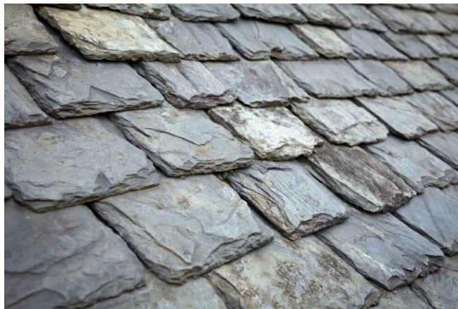
Figure 25 Slate Roof
