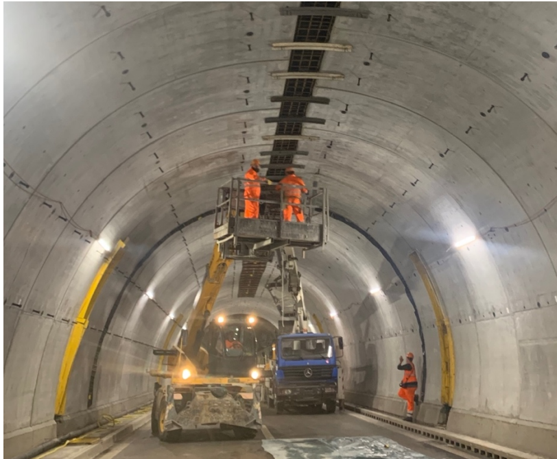
Figure 3.3-5 – Work in progress: 4 th step concrete injection
