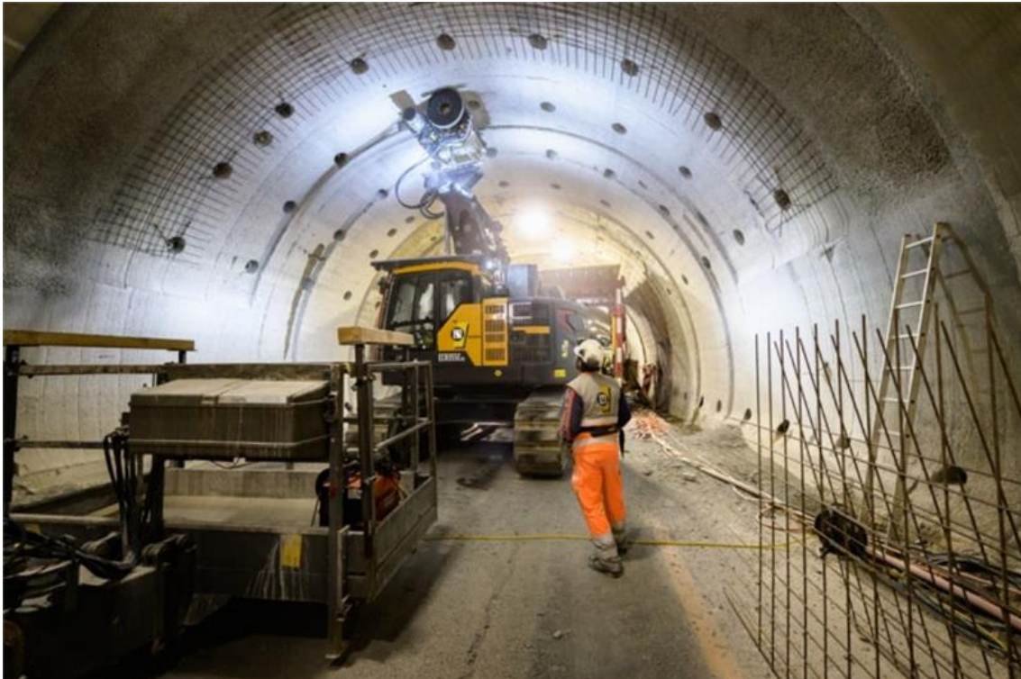
Figure 2.3-1 – FEDRO Tunnel: milling of the old lining
