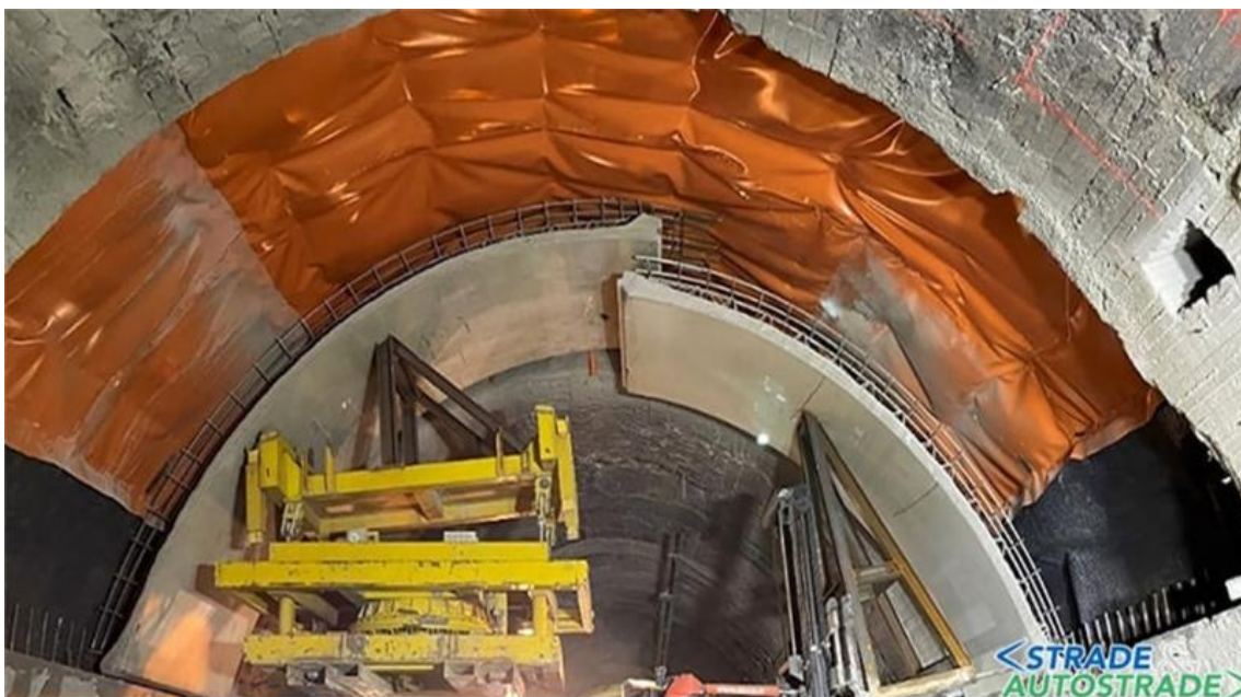
Figure 3 – Monte Galletto Tunnel: slabs installation and waterproofing sheets
