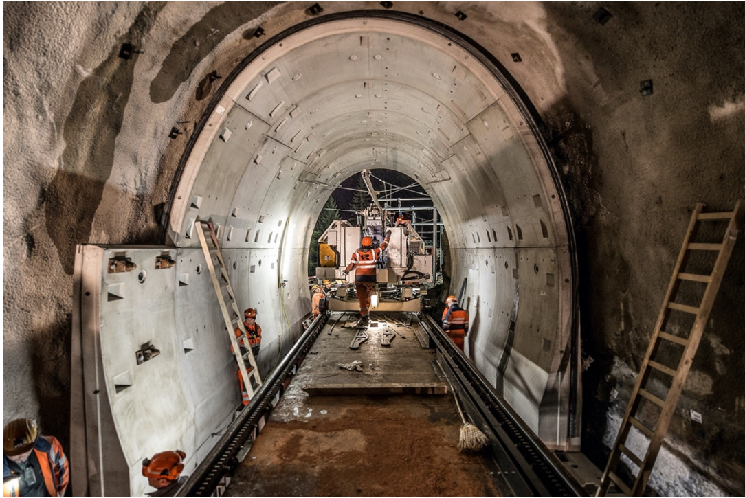
Figure 2.4-2 - Gletschera Tunnel: segments installation
