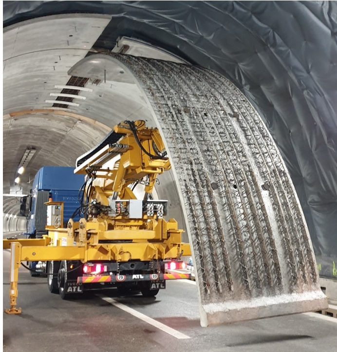
Figure 3.3-2 - Work in progress: prédalles installation
