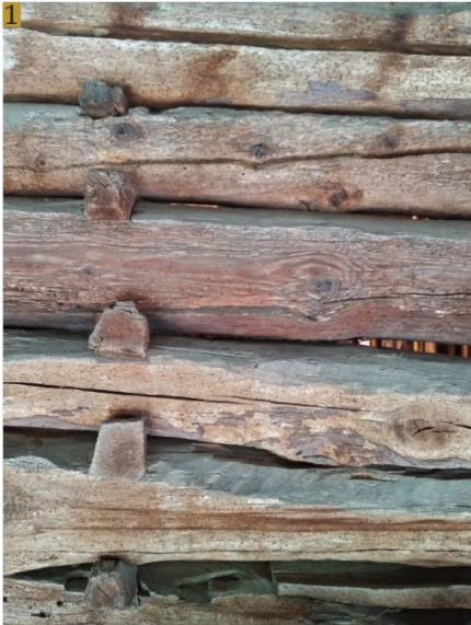
Blockbau structure in house in Alagna; made of larch and fir wood (Mirici Cappa, 1997)
