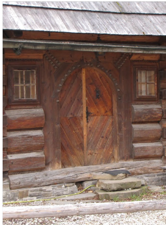
Entrance doors to house on Droga Do Rojów St., in Zakopane
