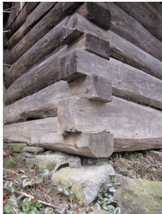
Figure 20 [left] Corner of a mountain hut in Strążyska Valley with visible rough foundation (photo Z.Miłek)
