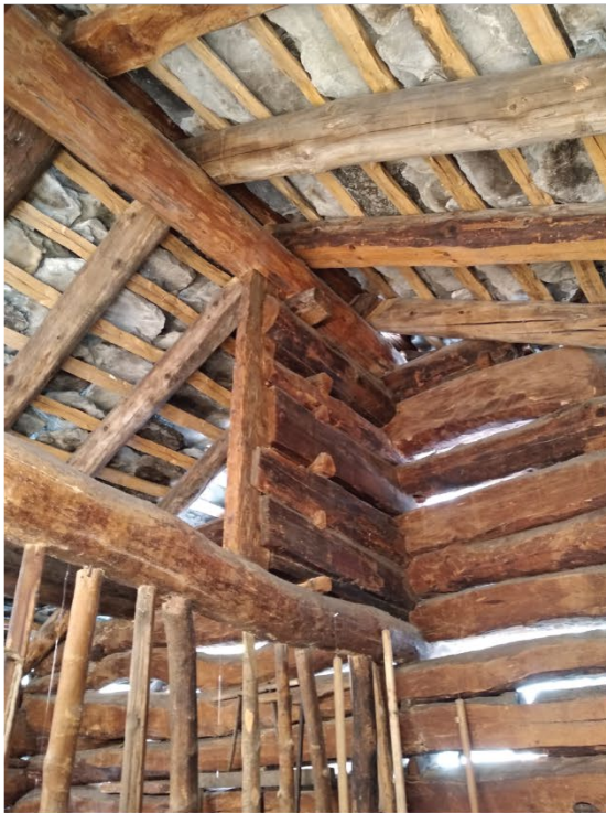
Carpentry of the roof (Remacle & Danilo, 2014)
