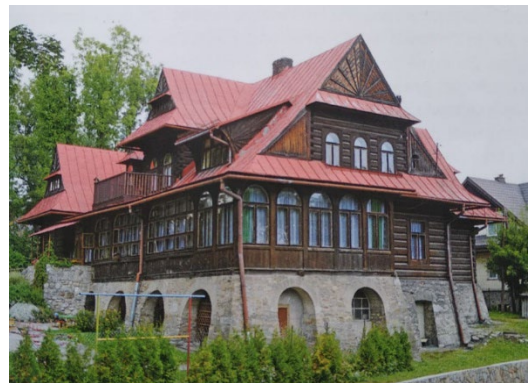
Figure 42 During the interwar period roof cover was changed to metal sheets, following the colour of the original design.
