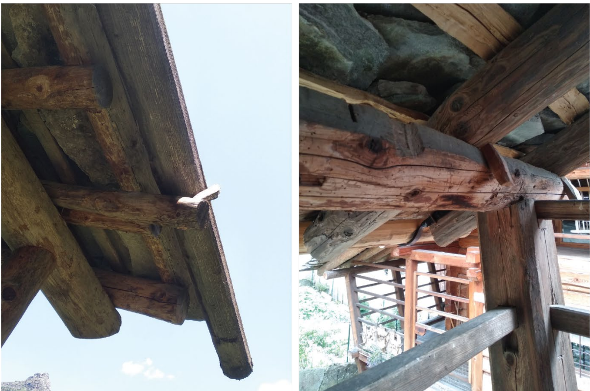
details of roof; houses in Alagna(photo: Z.Miřek)
