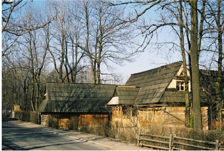
Figure 16 Podhale homestead from the 19th century (photo: J.Łaś)
