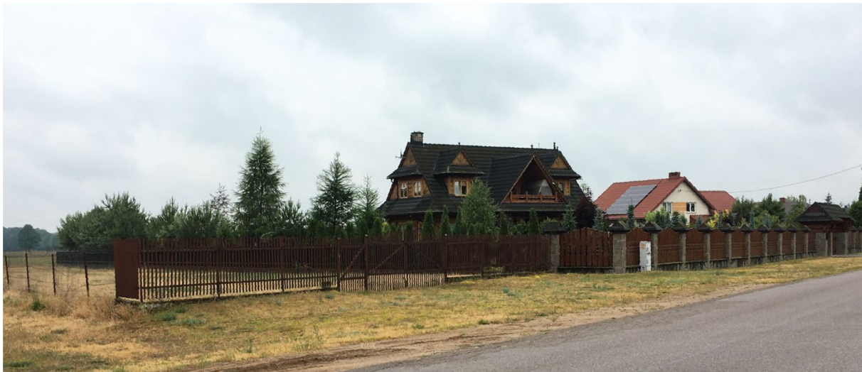
Figure 60 House built around 2010 - reinterpretation of Zakopane Style in Mazovia Voivodeship, central Poland, Kobylin (photo: Z.Mitek)
