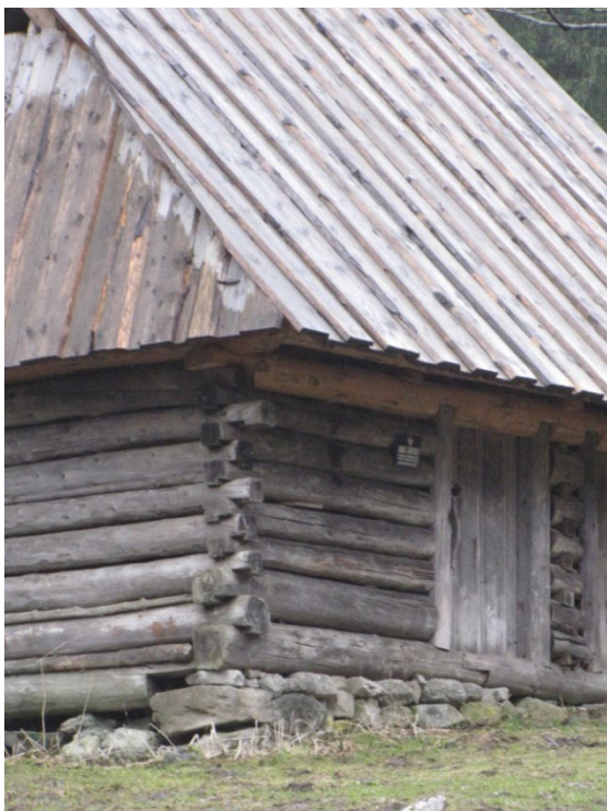
Figure 20 [left] Corner of a mountain hut in Strążyska Valley with visible rough foundation (photo Z.Miłek)
