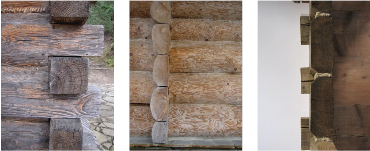
Figure 23 Apart from division shown on previous page there could be distinguish different types of plaza shape – some of logs were shaped with leaving rounded edges, others were formed to sharp edges
