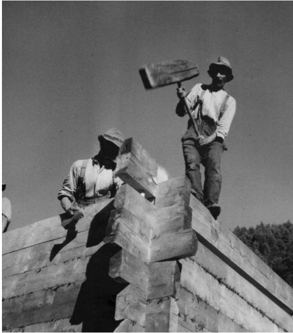
Figure 87 (left) Builders raising the blockbau wall, Vallese ,1930 (photo: Ernst Brunner)
