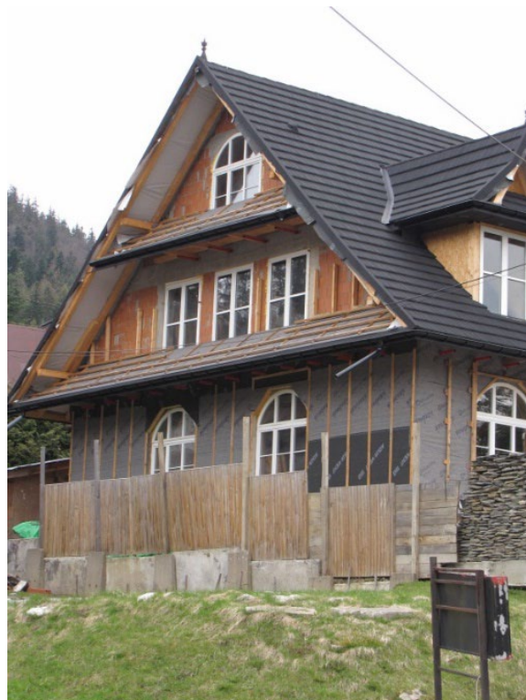
Figure 61 [left] interlocking planks on elevation; Zakopane (photo: Z.Miłek)
