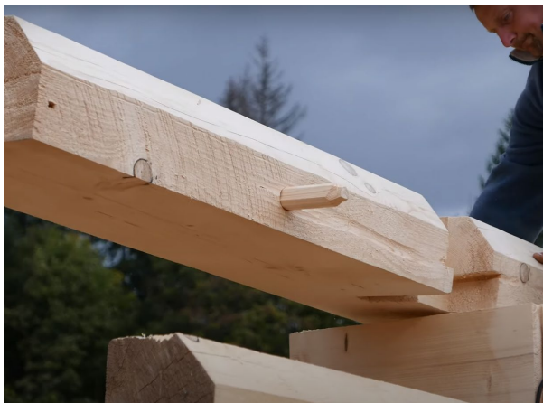
Figure 24 Peg installation (source: Studio 51 - biuro architektoniczne)
