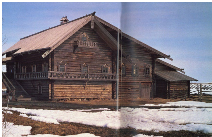
Figure 55 Yelizarov house re-erected in Kizhi (Opolovnikov et al. 1989)
