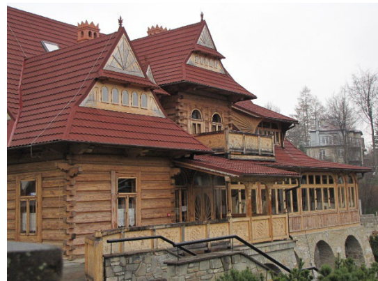
Figure 43 Villa after modernization conducted in 2017-18. The roof cover is in colour and shapes similar to the original project, but the material is different - metal sheets.
