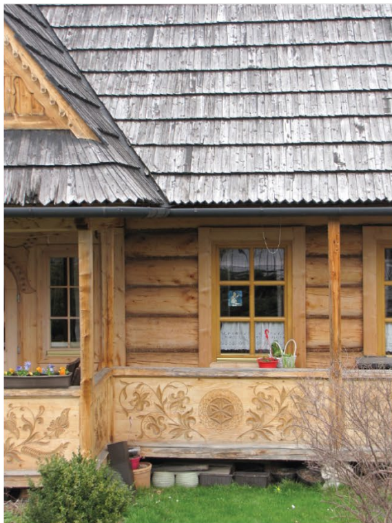
In the photo, the corner of the roof is circularly shaped - owijka
