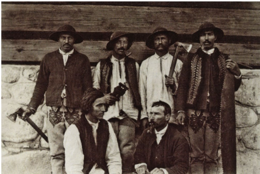
carpenters workers during construction of Villa "Koliba" in 1893 (Moździerz, 2020)
