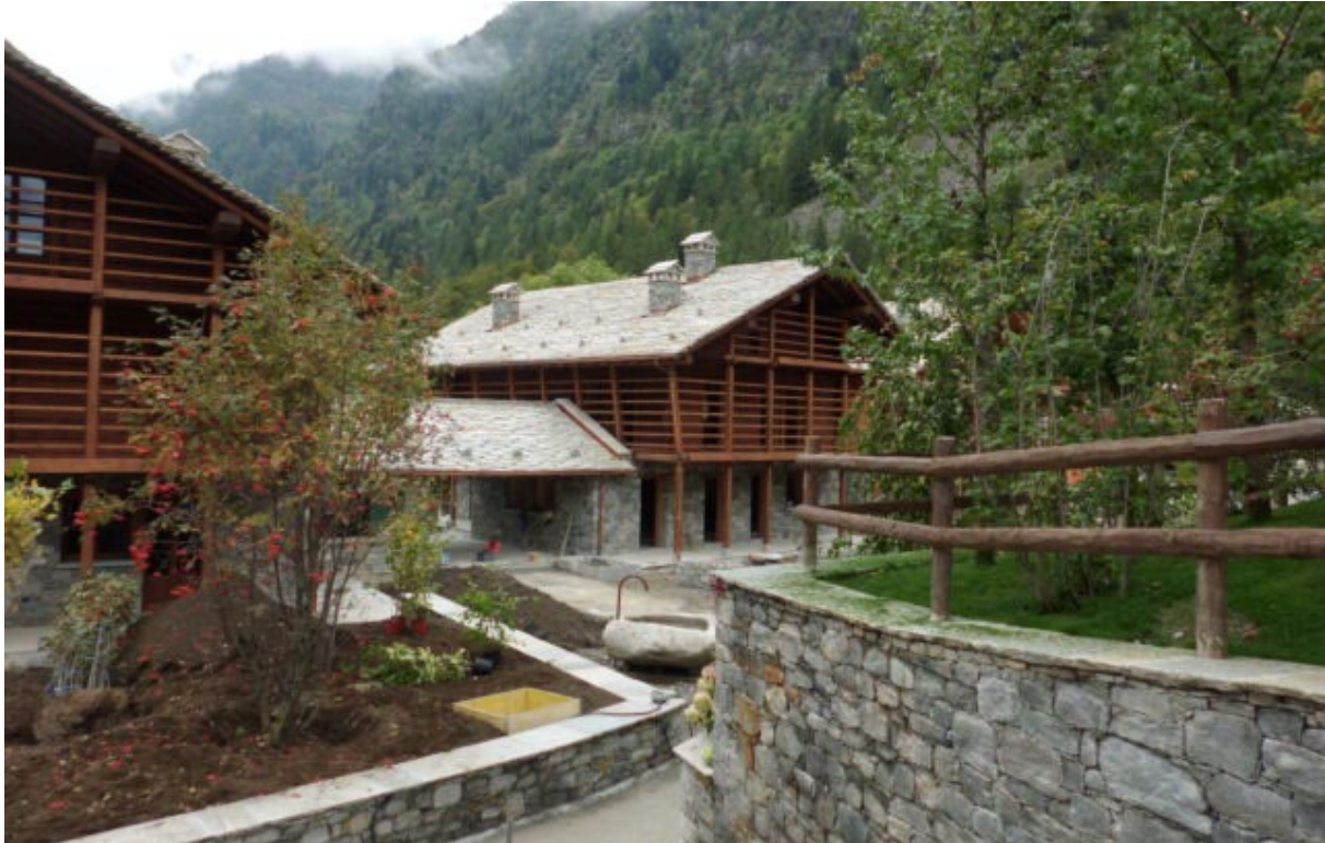
Figure 105 Newly risen residential buildings “Baite Monte Rosa” that follow the Walser tradition (source: https://www.illen.it )
