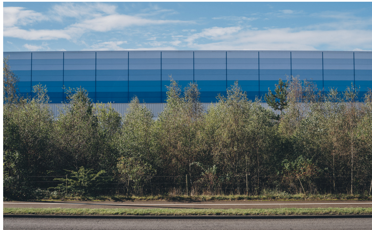
The exterior of Amazon Fulfillment Centre BHX1, Rugeley © Ben Roberts
