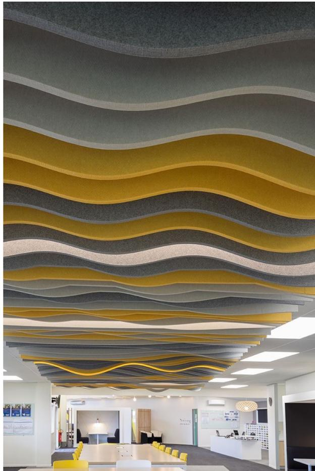
Figure 2 *Example of acoustic suspended baffle ceiling*
