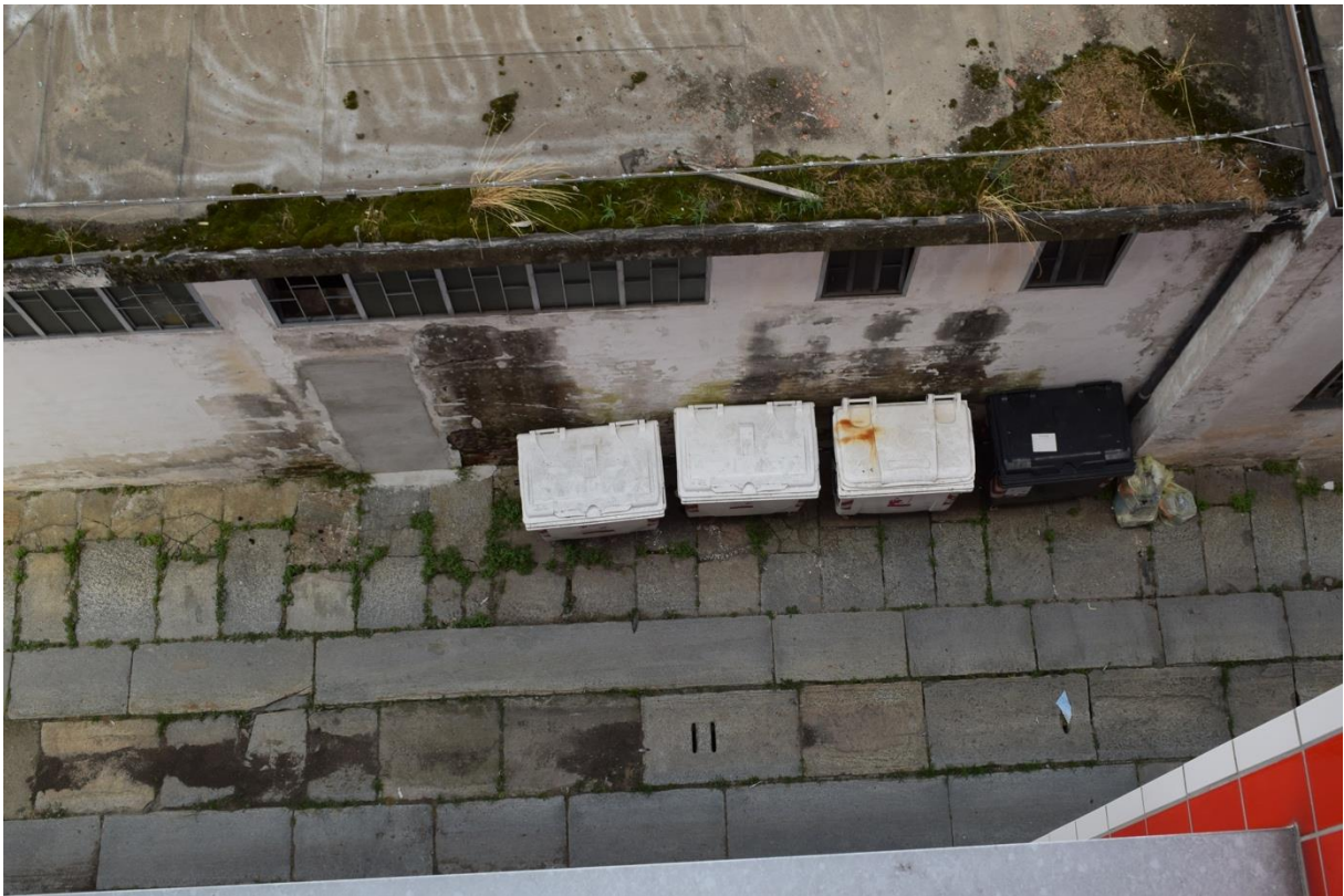
Figure 55 - Detail of the flooring of the internal viability.
