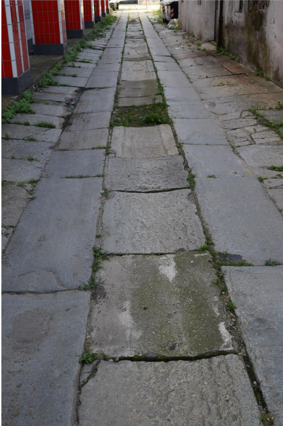
Figure 53 - Detail of the flooring on the internal viability.
