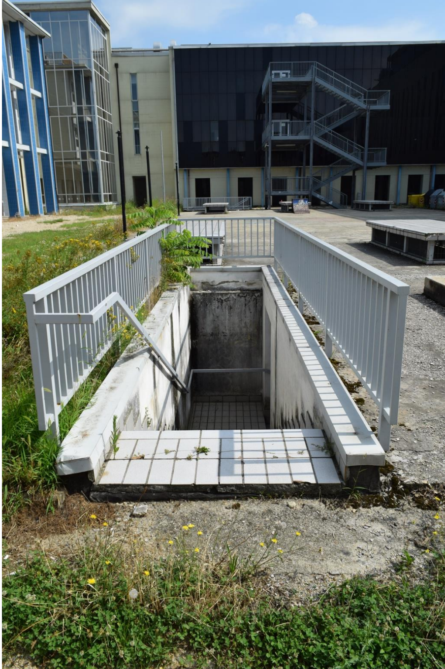
Figure 42 - Detail of the staircase to access the underground parking.
