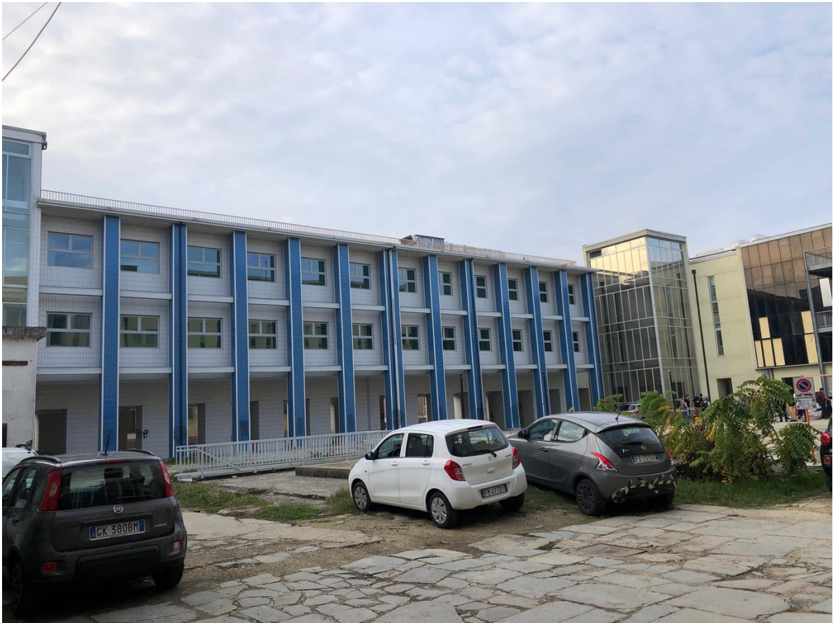
Figure 41 – View of the internal courtyard surrounded by the school complex on the north-westside and part of the municipality building on the east-south side.
