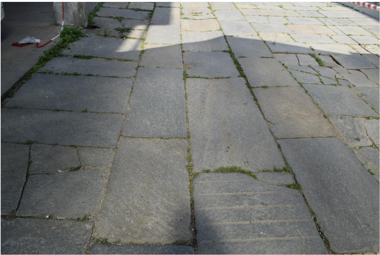
Figure 58 - Detail of the flooring near the historic entrance portal.
