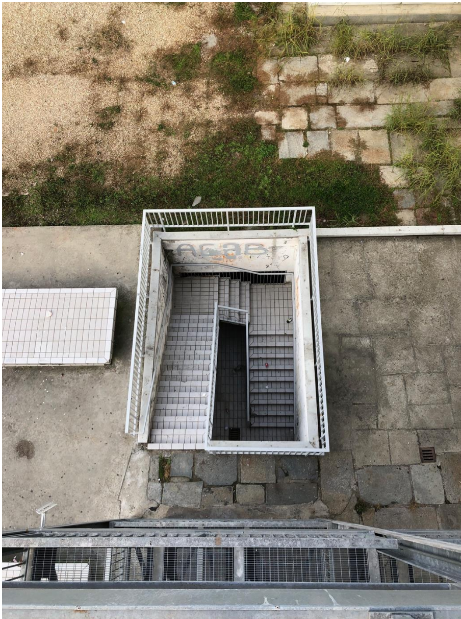
Figure 45 - Detail of the staircase to access the underground parking. Picture taken from the top of the emergency staircase of the school.
