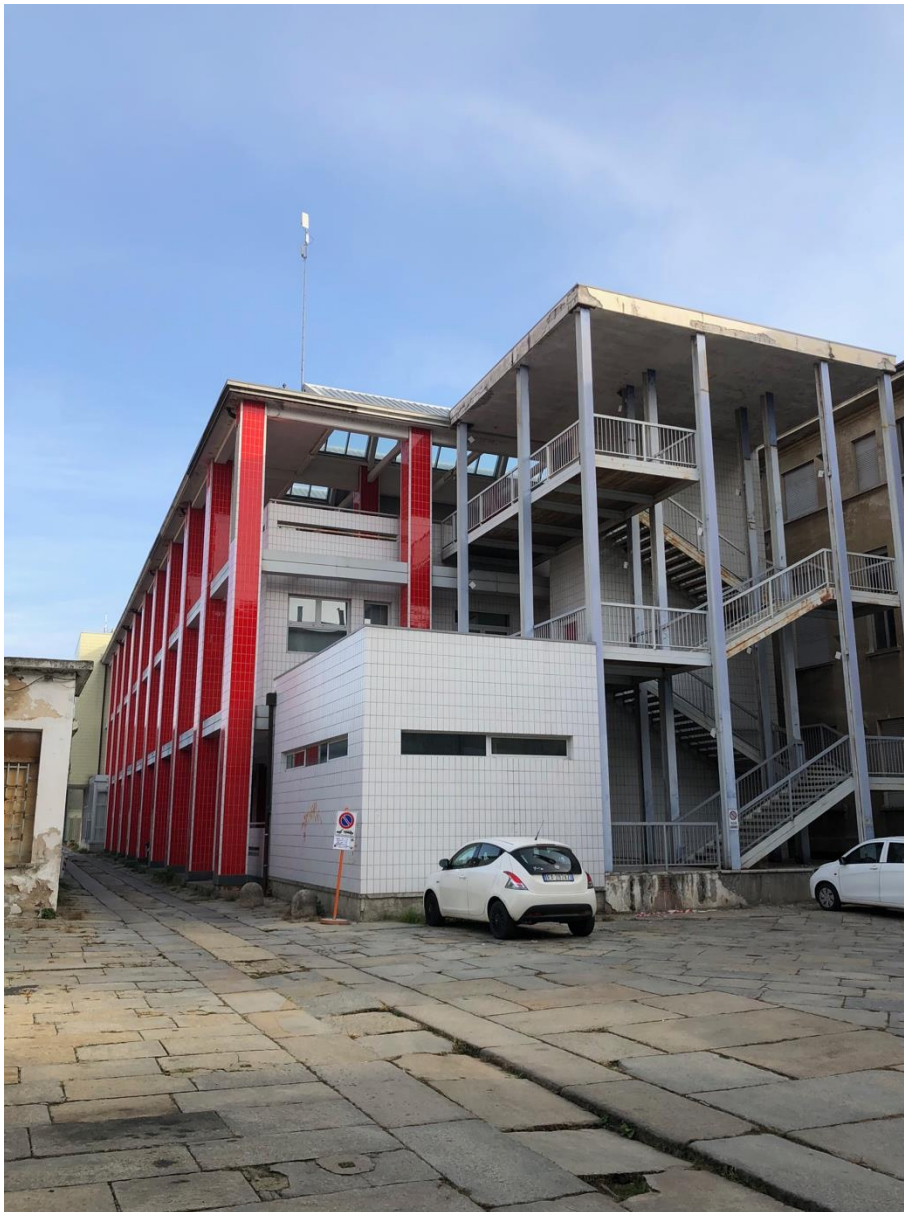
Figure 38 – View of the internal viability in between the current municipality building on the right and the former weaving building on the left.
