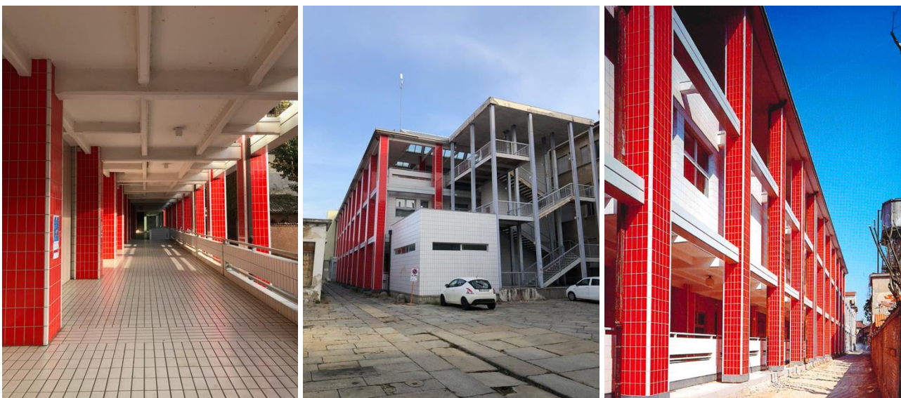
Figure 20 – Views of the refurbished complex. From left to right: the ground floor walkway, view from the inner courtyard and view of the building on via Frichieri.
