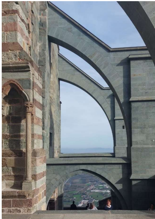
Figure 40 - Flying buttress system, build by d'Andrade Source: Marina Boschetti (2022)
