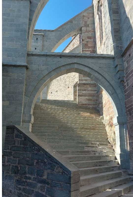
Figure 39 - Flying Buttress by d'Andrade Source: Marina Boschetti (2023)
