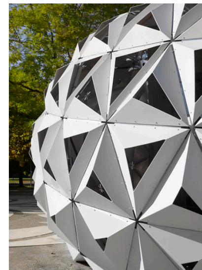
Figure Bp11: ArboSkin Bioplastic Façade Source: https://urbannext.net/
