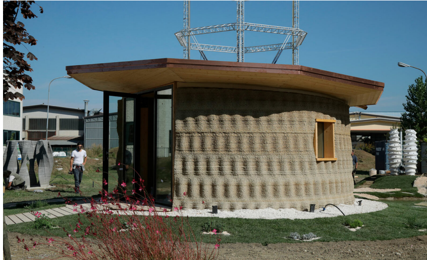
Figure Hk17-18: Gaia project and 3D printing construction process - by Rice House Source: https://www.ricehouse.it/
