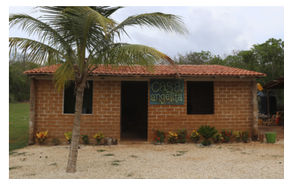
Figure Sw20: Casa Angelita - (MX) first home built with Sargablocks
