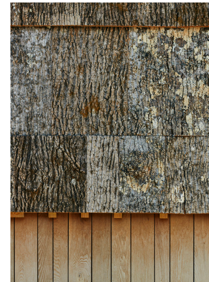
Figure Ck21: Poplar grove - In the alleys - by BLDUS Architects - bark cladding Source: https://www.archdaily.com/995031/poplar-grove-bldus
