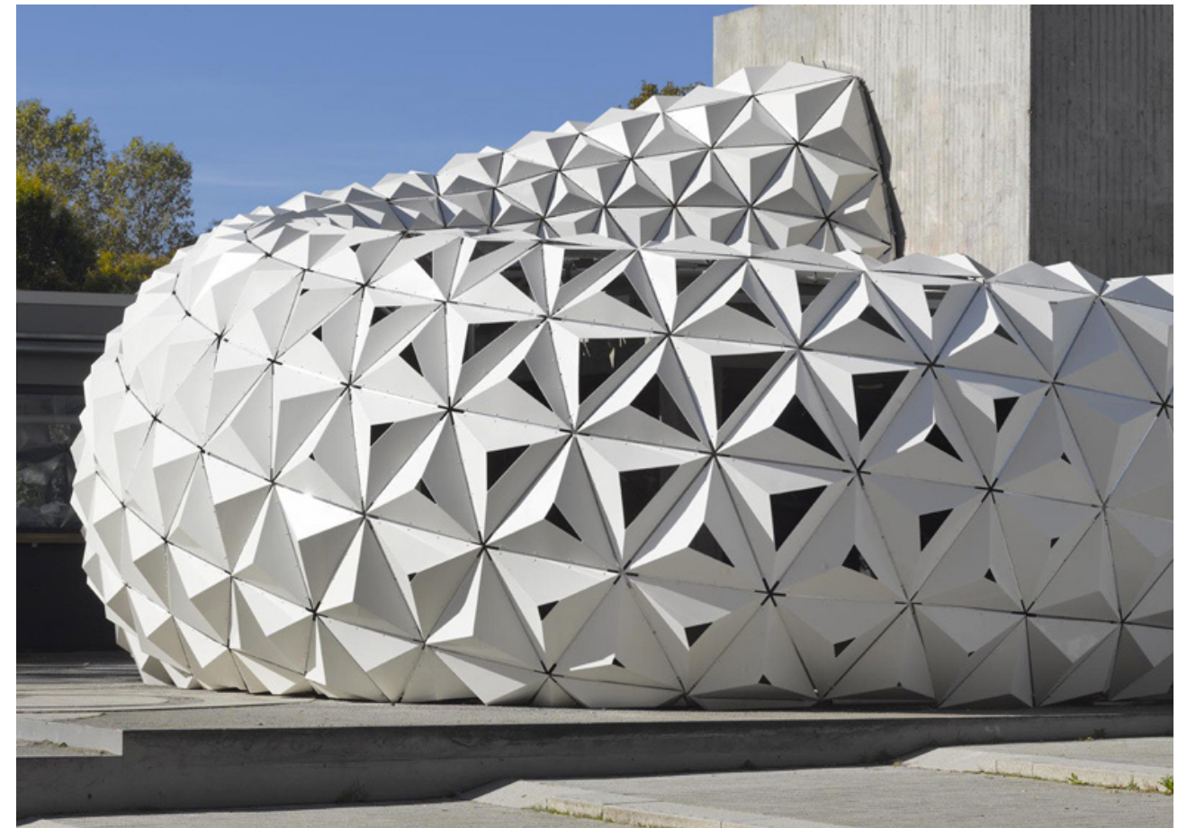
Figure Bp10: ArboSkin Bioplastic Façade Source: https://urbannext.net/
