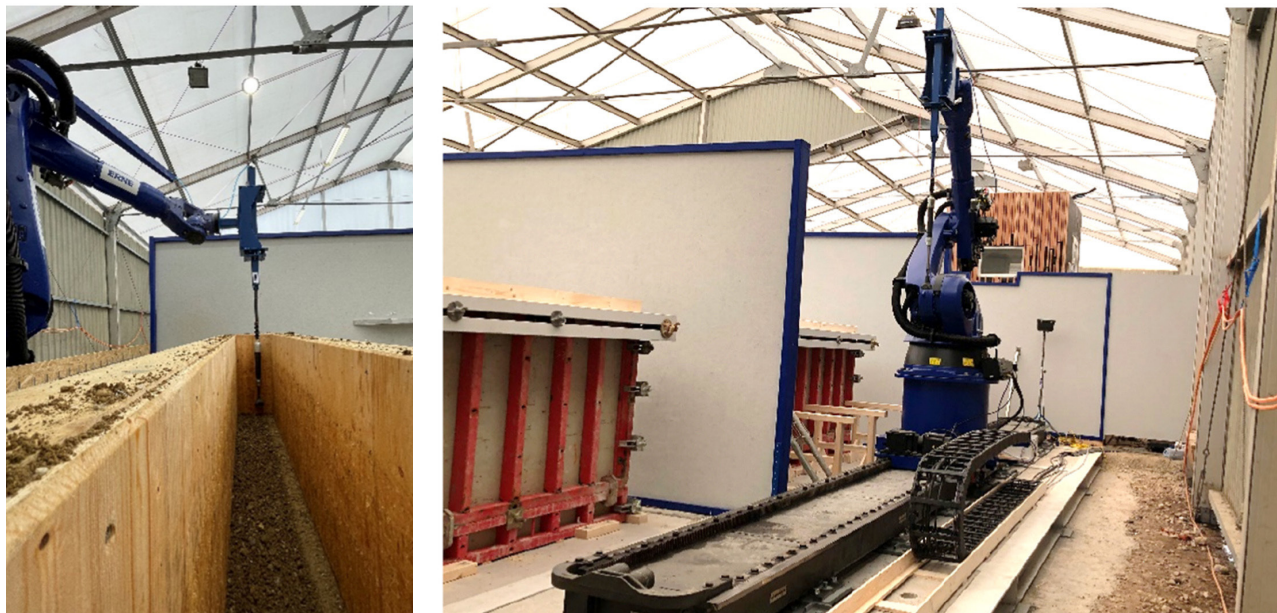
Figure 02.3.2: Robotic ramming system by ERNE Source: Mohamed Gomaa, Sascha Schade, Ding Wen Bao, Yi Min Xie, Automation in rammed earth construction for industry 4.0: Precedent work, current progress and future prospect, Journal of Cleaner Production , Volume 398, 2023, 136569, ISSN 0959-6526, https://doi.org/10.1016/j.jclepro.2023.136569
