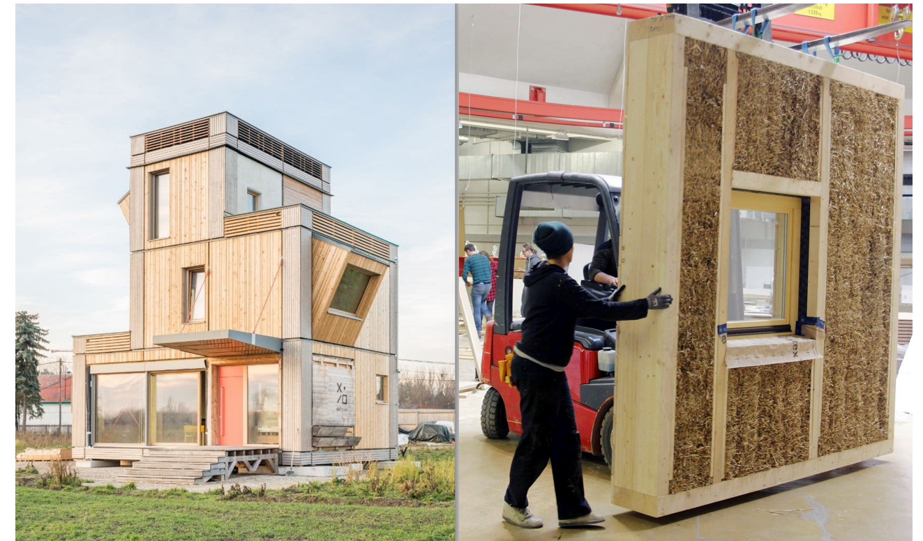
Figure St15: Image of the Vivihouse project and the wall straw prefabricated wall panels Source: https://www.vivihouse.cc/
