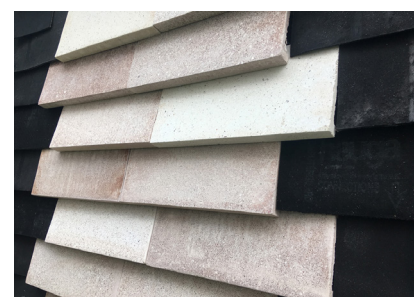
Figure Ss08: Oyster hanging tiles Source: https://localworksstudio.com/projects/shellcrete-transforming-sea-shells-into-low-carbon-materials/
