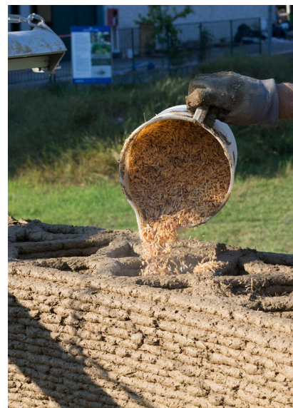
Figure Hk019-20: Wall 3D printing construction process and rice husk infill - by Rice House Source: https://www.ricehouse.it/
