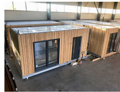
Figure 02.4.3: Wood modular construction Source: https://www.sipeurope.eu/en/se-sip-construction-system/using-sip-system/modular-buildings/
