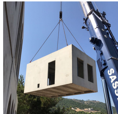
Figure 02.4.2: Concrete modular construction Source: https://megaprefab.com/
