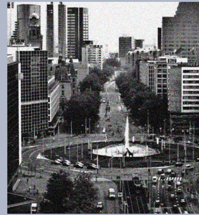
Finish of reconstruction
