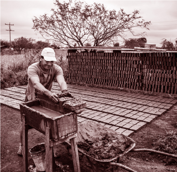
Figure 14. Construction industry. (Padron,2022)
