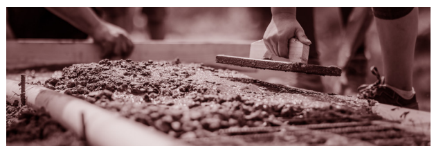
Figure 12. Construction field. (Quiros,2019)
