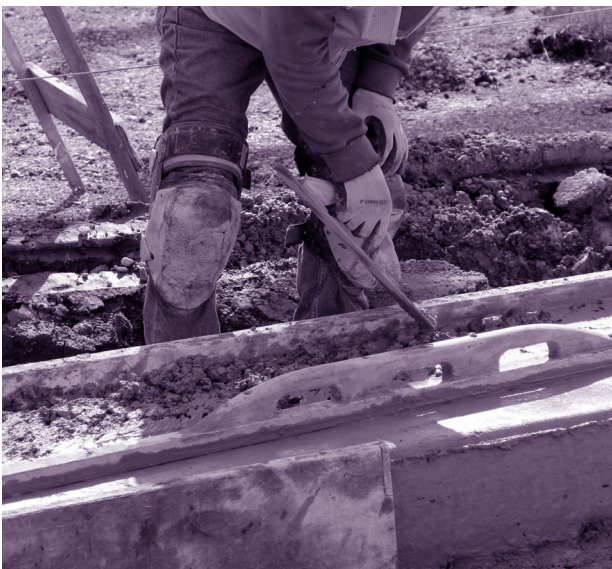
Figure 5. Construction materials. (Pexels, 2020)
