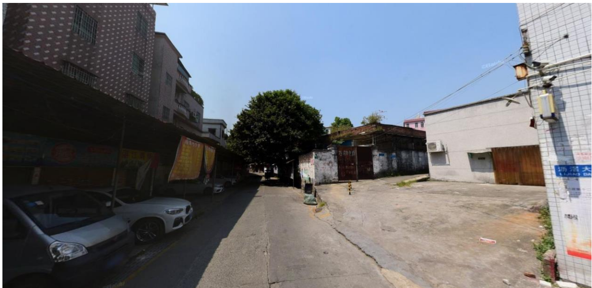
Figure 5-39 Original street view of Lijiao Dashi Street (source: Baidu Street Map)
