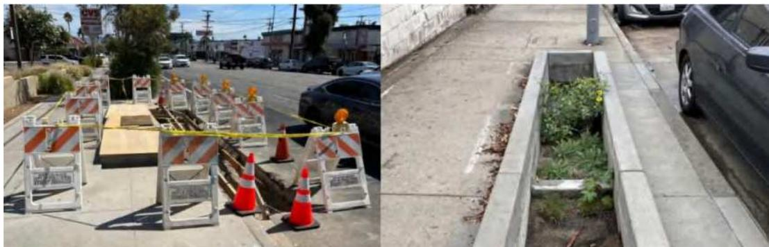
Fig. 3-3 Installation of bio-pit rain gardens(Source: SFMTA)
