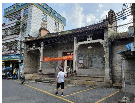
Fig. 4-22 Street view of Shiya Wei Clan Ancestral Hall(Source: Photo by author)
