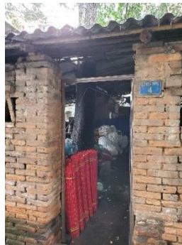
Fig. 4-10 Brick building (Source: Photo by author)
