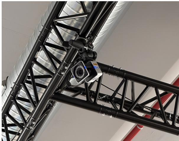
**Figure 4.2:** Truss System for Vicon Cameras.
