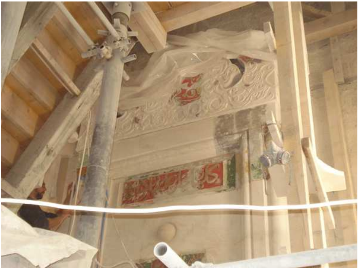
Anastylosis and reconstruction of missing parts of the mihrab in the mosque "Ferhadija" in Banja Luka
