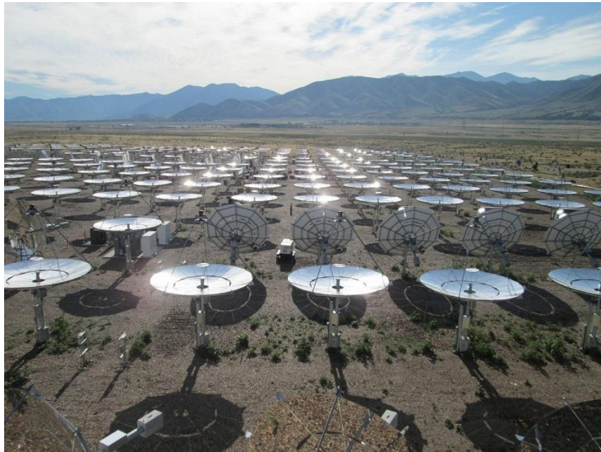
Figura 2.23 – Impianto SPD, Tooele Army Depot [31]
