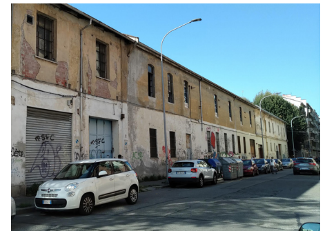
Abandoned building in Aurora, Turin. Via Aosta Source: Google Earth
