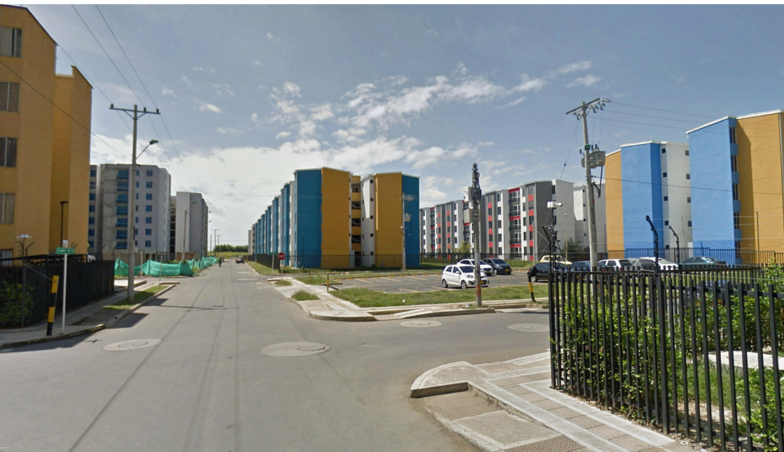
Horizontal growth at Cali, Colombia. Source: Google Earth.
