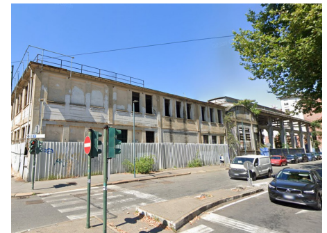
Abandoned building in Aurora, Turin. Via Bologna Source: Google Earth
