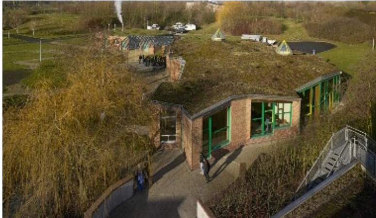
Figure 3.12. View of the green roof of the building ( https://www.architectural-review.com . 2023)
