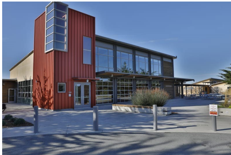
Figure 3.14. View of the large windows in the classrooms of the school building (www.chartwell.org 2023)
