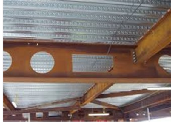
Figure 5.35. Solid and open web steel beams ( http //images.google.com )
