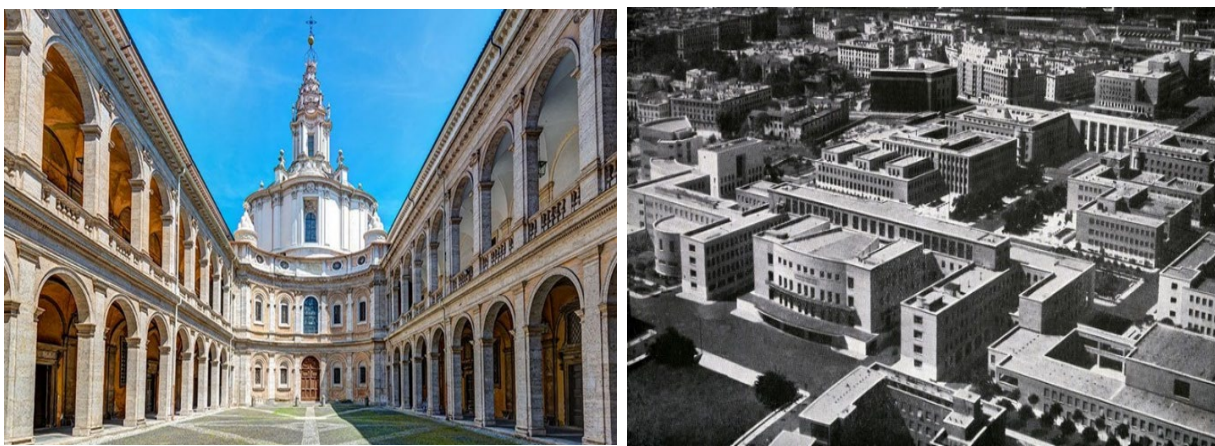
Figure 2.5. View of the courtyards in the old and new buildings of La Sapienza ( https://pavaedu.com/roma-la-sapienza-universitesi )
