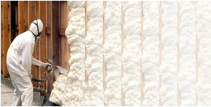
Fig 3.10 Spray foam insulation during installation
