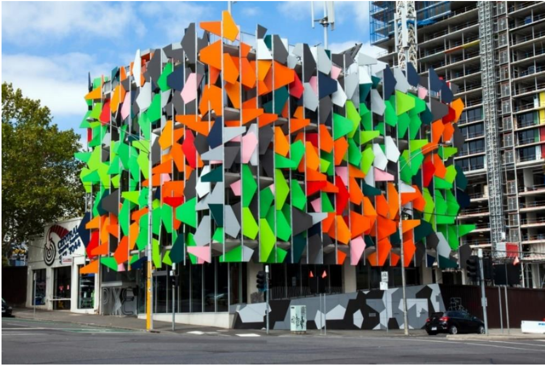
Fig 2.7 Pixel building view (Façade)
