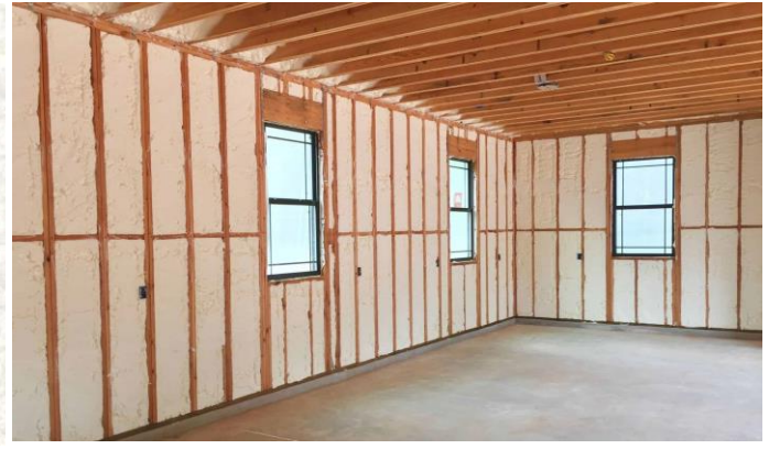
Fig 3.11 Spray foam insulation after Installation
