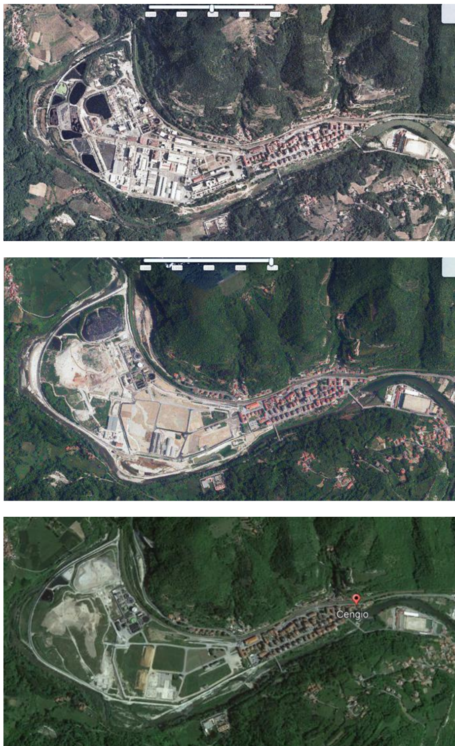
Figure 38. Comparison between the state of the former ACNA site of Cengio in 2000 (above), in 2012 (central) and 2016 (below)
