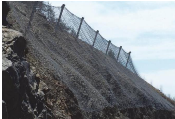
Figura 23 Barriera ibrida da 3.000 kJ — Route 248, Lehigh Gap, Lehigh Township, Pennsylvania, Stati Uniti (6)
