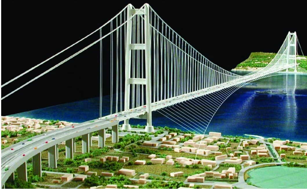
Figure 1.18 Additional cable system
