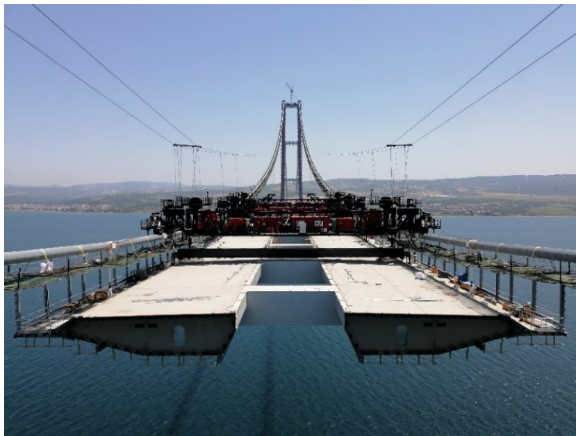
Figure 1.4 View of the Canakkale bridge during its construction [3]
