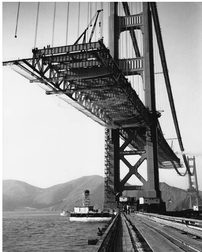
Figure 1.2 View of the Golden Gate bridge during its construction
