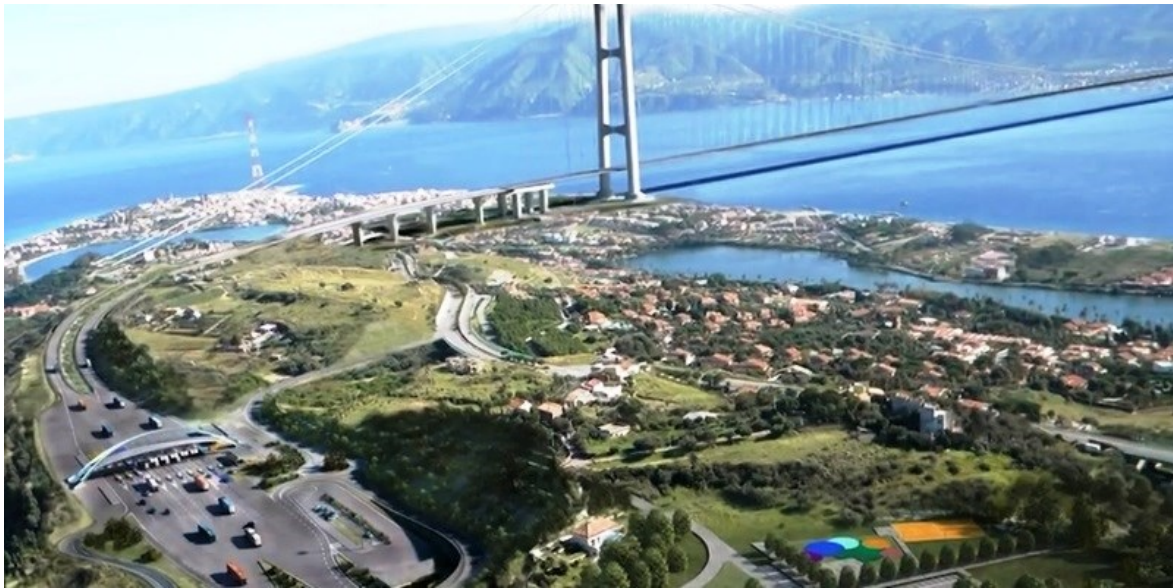
Figure 4.6 Lateral span on Sicilian side
