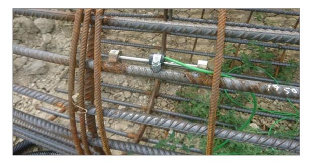
Figure 2.3 Vibrating wire gauges embedded in RC (gestecno.it)
