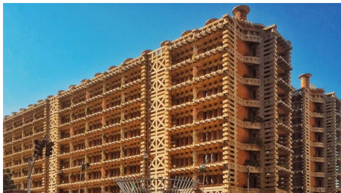
Figura 28: Eastgate building centre di Harare, in Zimbabwe
