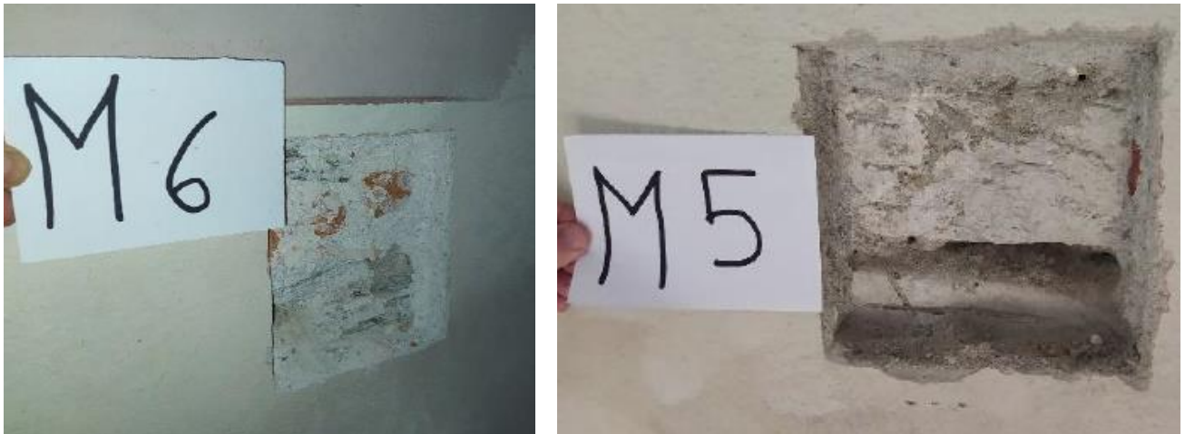
Figure 1-32. View of the test area - M5 and M6.
