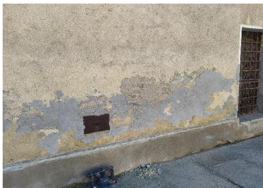
Figure 1-31. View of the test area - M4
