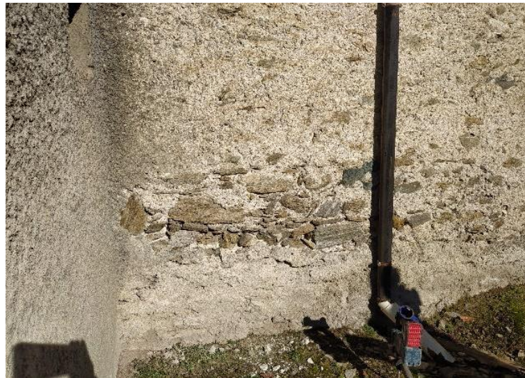
Figure 1-29. View of the test area - M2.
