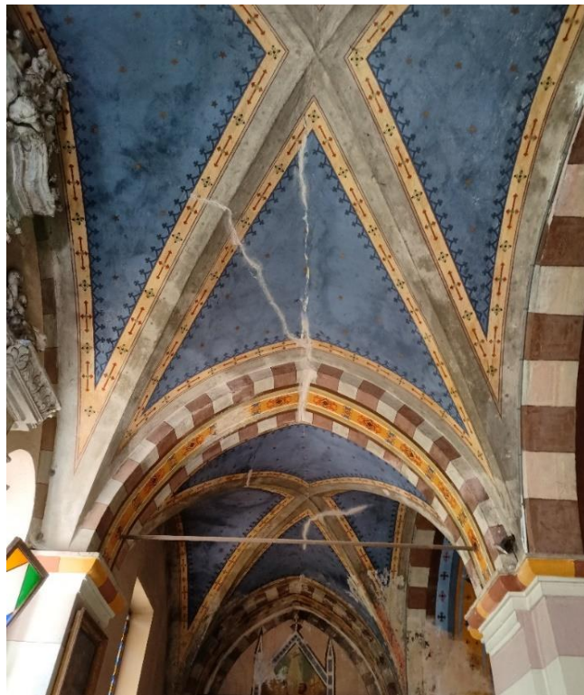
Figure 1-9. Groin vault located in one of the lateral aisles.
