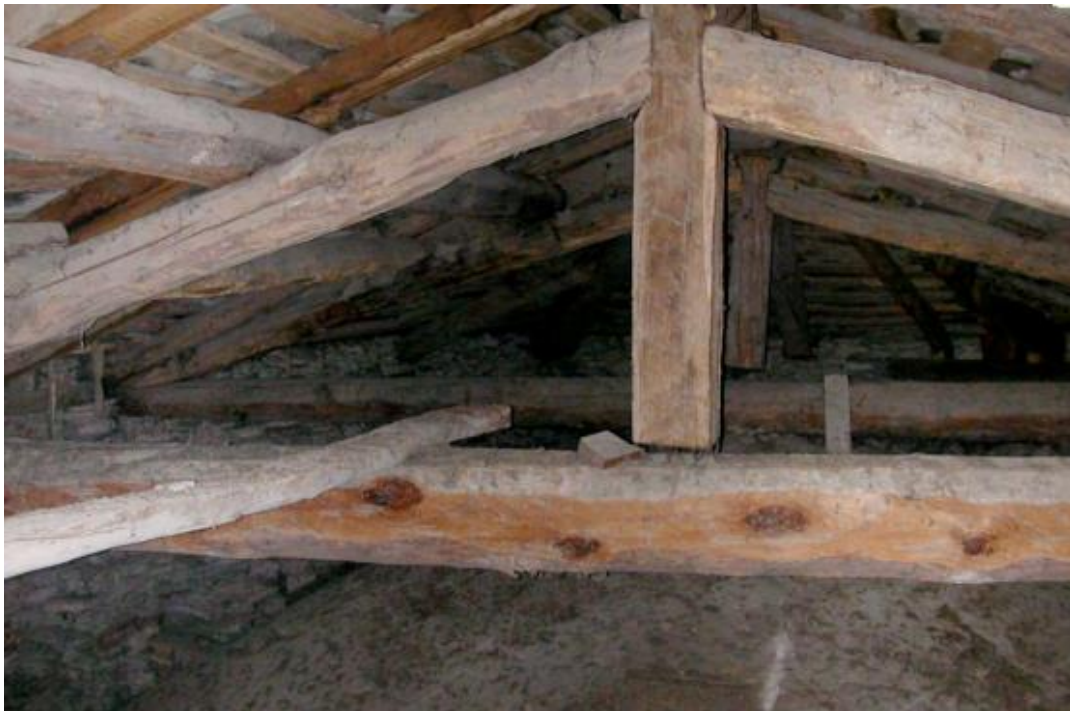
Figure 1-15. Condition of the roof.
