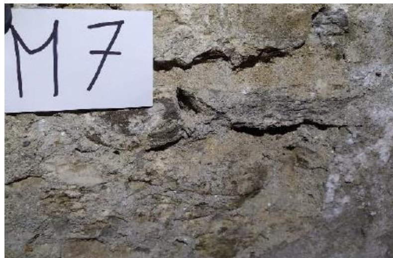
Figure 1-33. View of the test area -M7.
