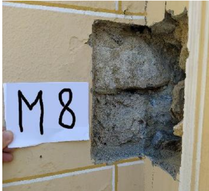
Figure 1-34. View of the test area -M8.
