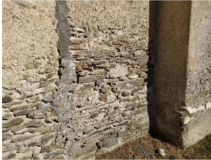
Figure 1-28. View of the test area – M1.
