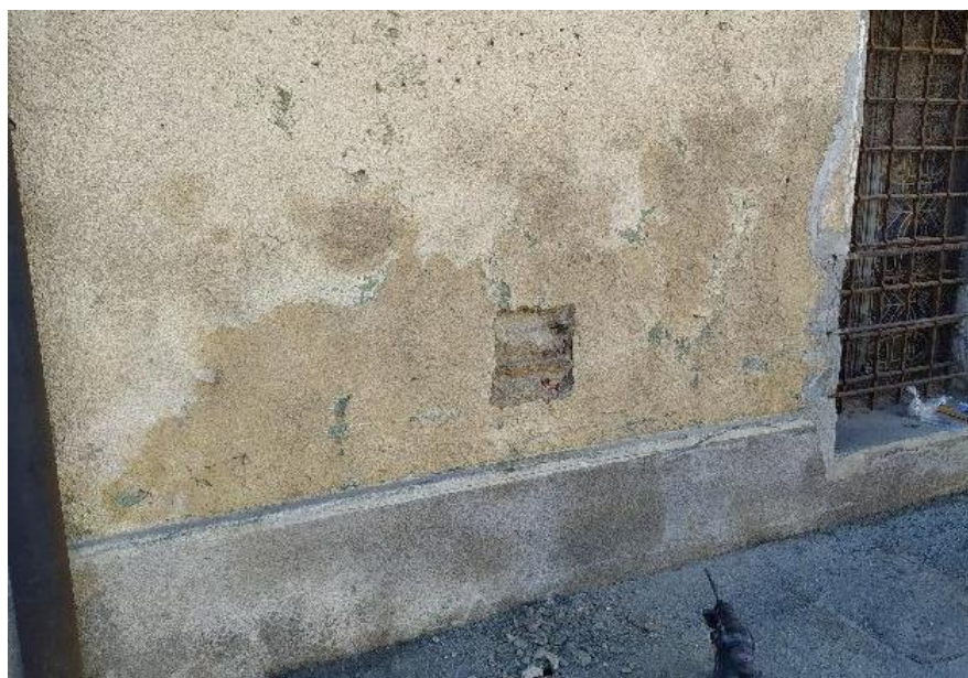
Figure 1-30. View of the test area - M3
