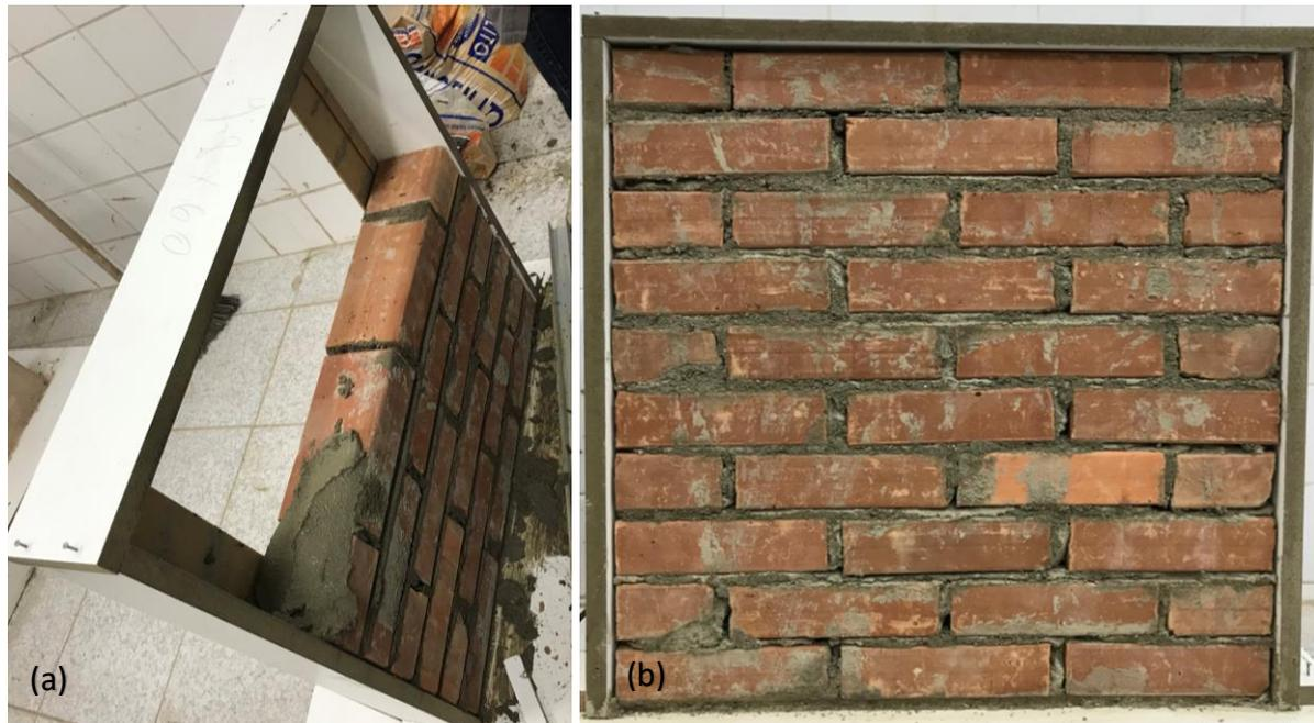
Figure 5.2 - Brick wall during construction (a); fully constructed (b)
