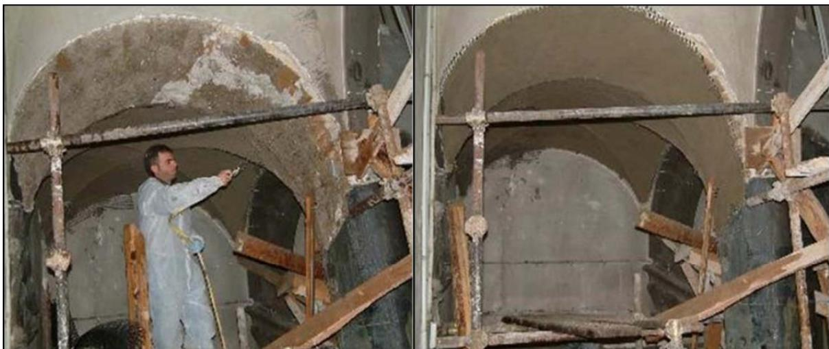
*Figure 2.3 - Masonry vault intradoxal strengthening with AR Glass fiber grid & mortar [3].*
