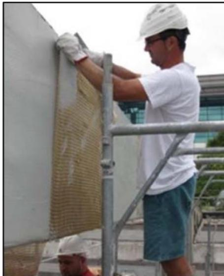
*Figure 2.5 - Beam shear strengthening with PBO fiber grid embedded in mortar [3].*
