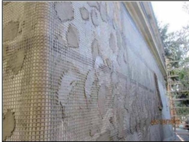
*Figure 2.1 - Basalt textile grid application on masonry wall [3].*
