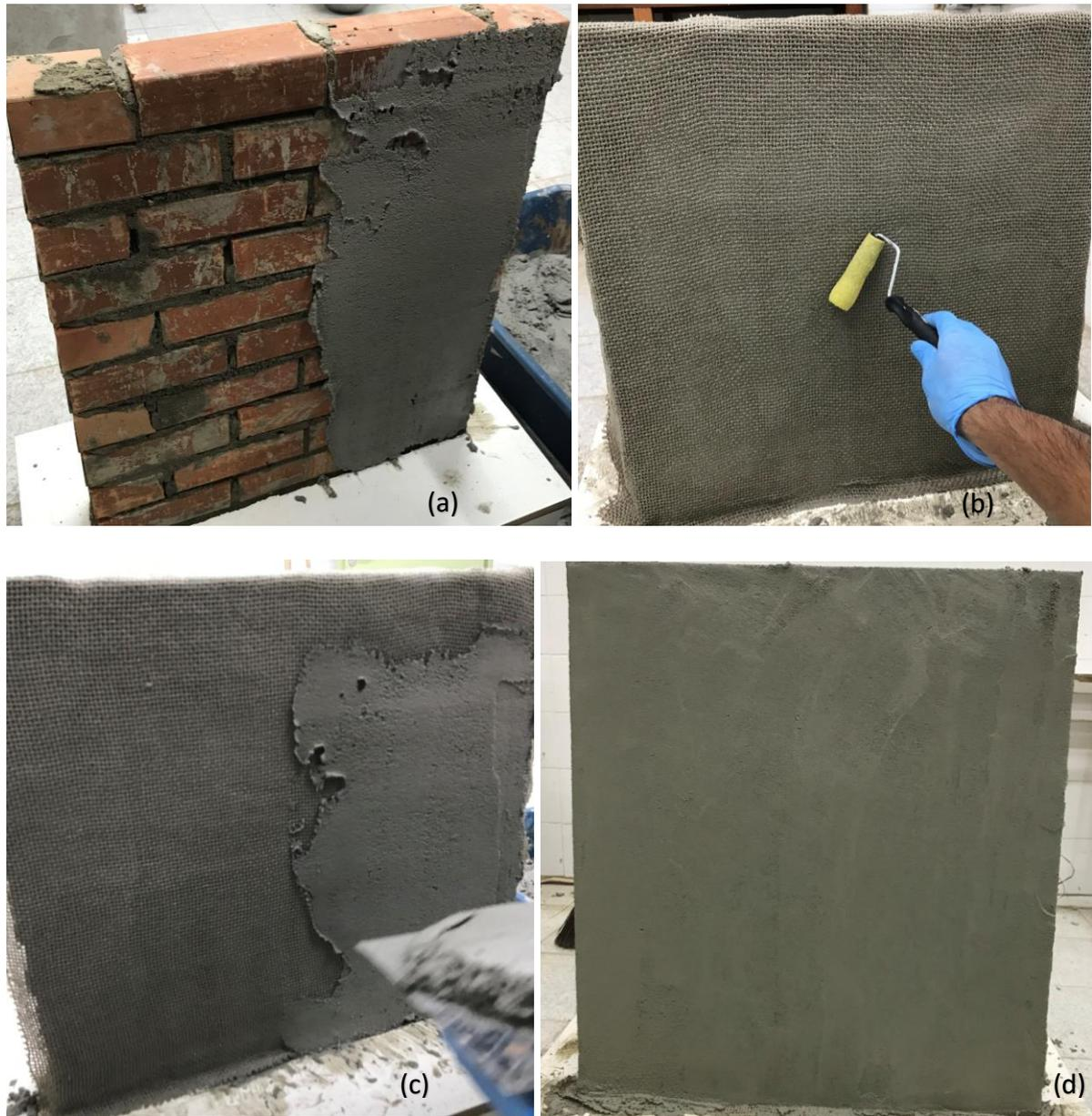
*Figure 5.3 - Application of 1st mortar layer (a); embedding of flax-fabric (b); application of 2nd mortar layer (c); smoothed final assemblage (d)*
