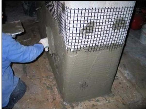
*Figure 2.4 - Column confinement with AR Glass fiber grid & mortar [3].*
