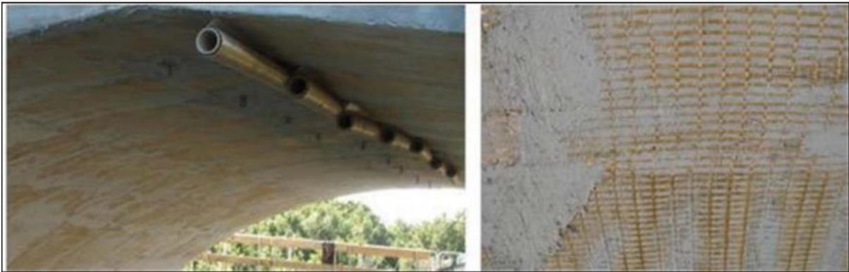
*Figure 2.2 - PBO mesh used for intradoxal strengthening of concrete arch bridge [3].*
