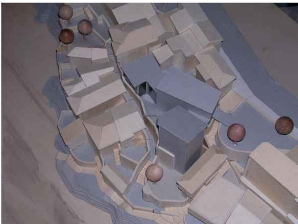
Part of the play school is inside existing derelict buildings and it is modelled inside this area in an “L” shape. The project consists of a tower and six floors joined by a foot-bridge to a lower and more massive central building. This building gives onto the main street Marsala Tita by a second foot-bridge. This is due to the fact that the play school is on different levels as the planned site slopes down towards the river Neretva.
