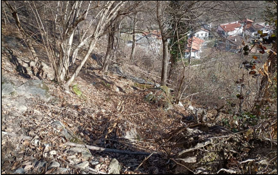
Figure 4-48 Site inspection following a series of detachments (from Dr. PGeol Chiuminatto)
