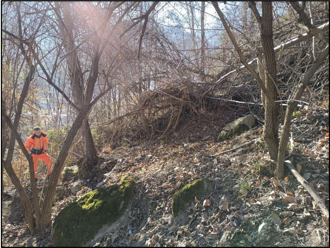
Figure 4-50 Site inspection following a series of detachments (from Dr. PGeol Chiuminatto)
