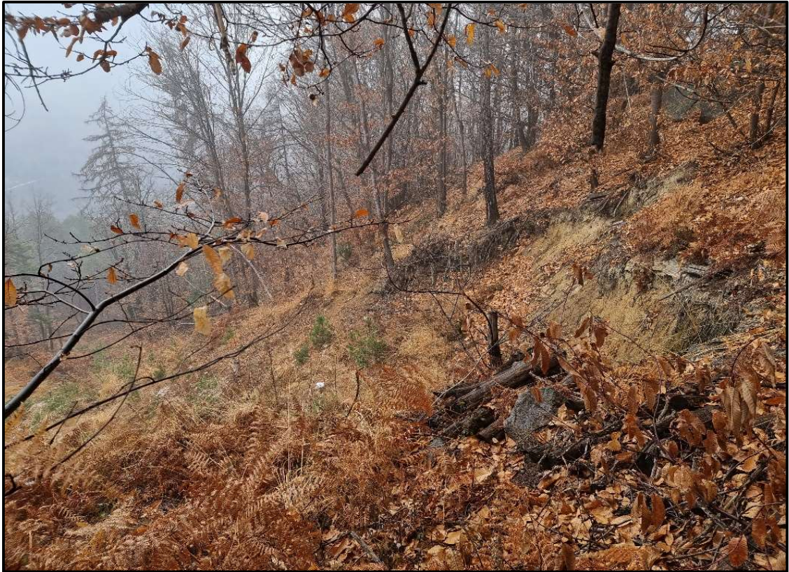
Figure 4-11 Current situation of the landslide detachment zone – View from above – Survey January 17, 2023
