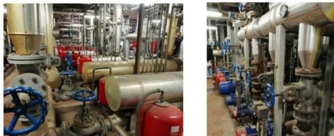
Figure 34 Heat Exchangers AEPAX (left) and pumps (right)
