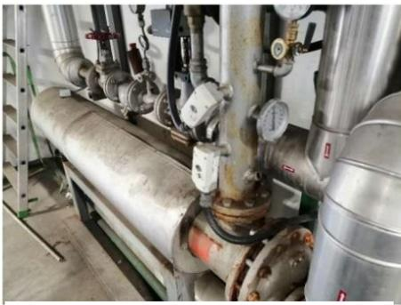
*Figure 29 Heat Hexchanger S.C.T.*
