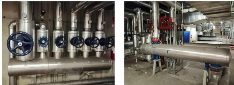
Figure 36 Collectors BHS (left), heat exchangers BHS (right)
