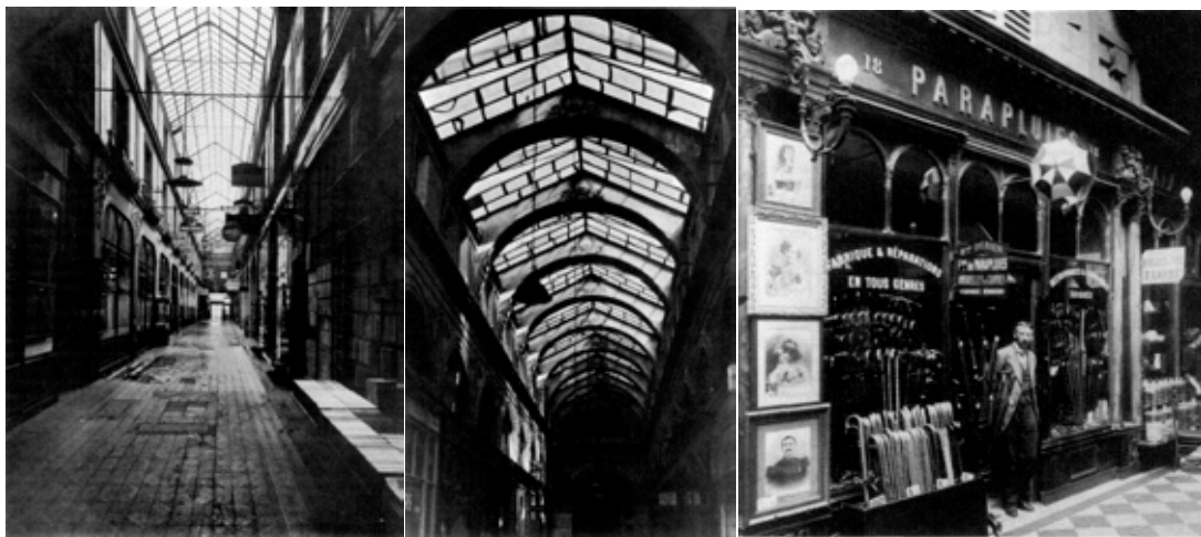
Fig.3-2. The Passage de l'Opera, glass roof and iron girders, shops in arcade of Paris
