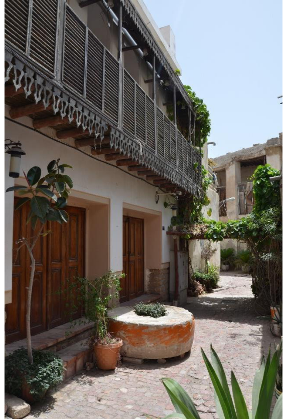
Figure 3-32: These wooden louvers, locally called Shanashil in city of Bushehr (Photo by Arsalan Chabok)
