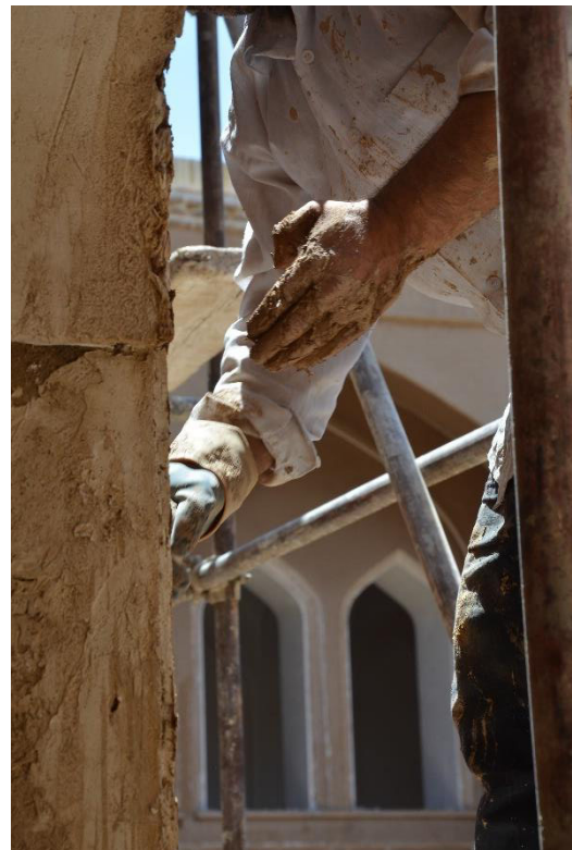
Figure 3-82: Mud walls are made of moist earth mixed with water and microscopic particles of straw. (Photo by Arsalan Chabok)
