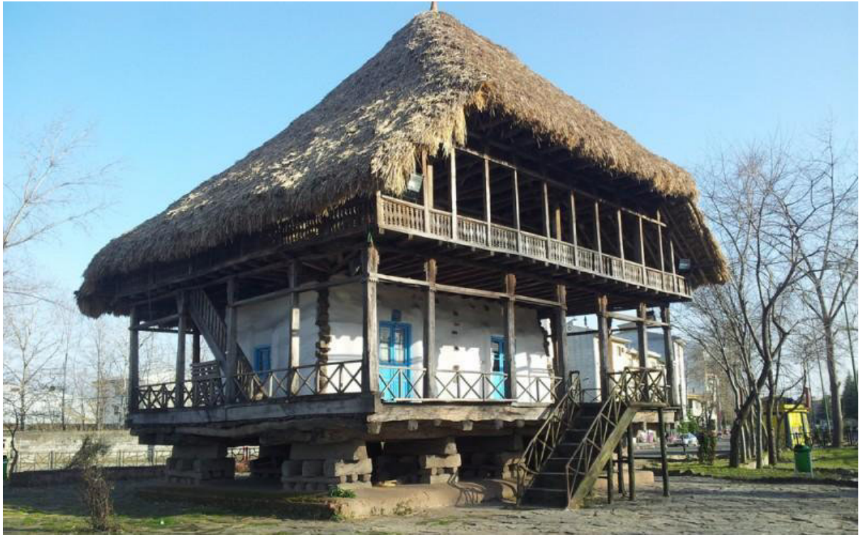
Figure 3-10: A typical house raised on wooden piers with two continuous balconies around and a thatched roof cover in the lowlands of the Gilan Province. (Photo by Maryam Gardoni)
