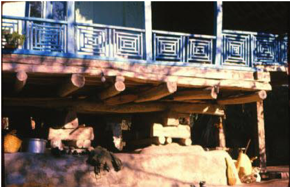
Figure 3-17: Details of wooden piers under a house near Langarud. (Photo by Vahid Ghobadian)
