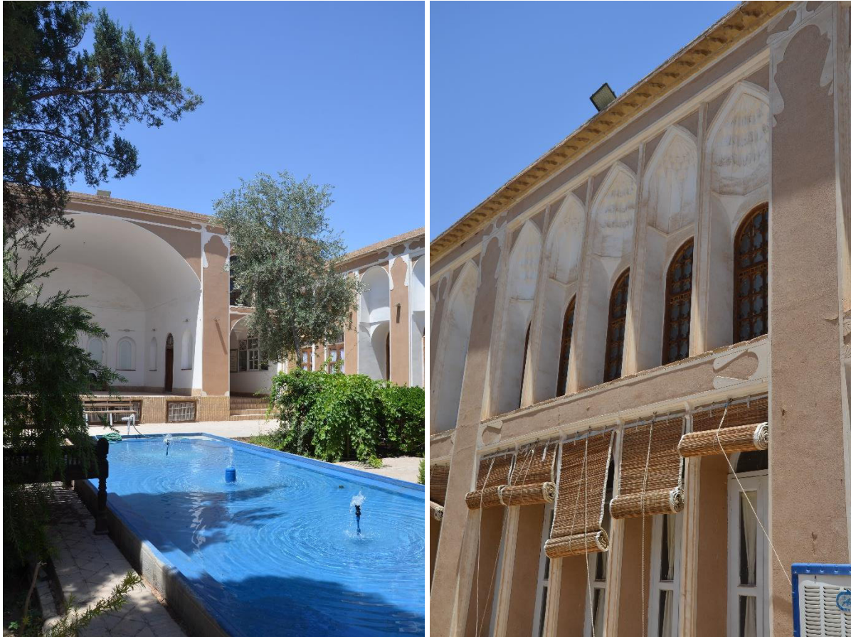
Figure 3-73: Summer building where is open and have windcatcher on top(left) and fall and spring area in two side (right). (Photo by Arsalan Chabok)
