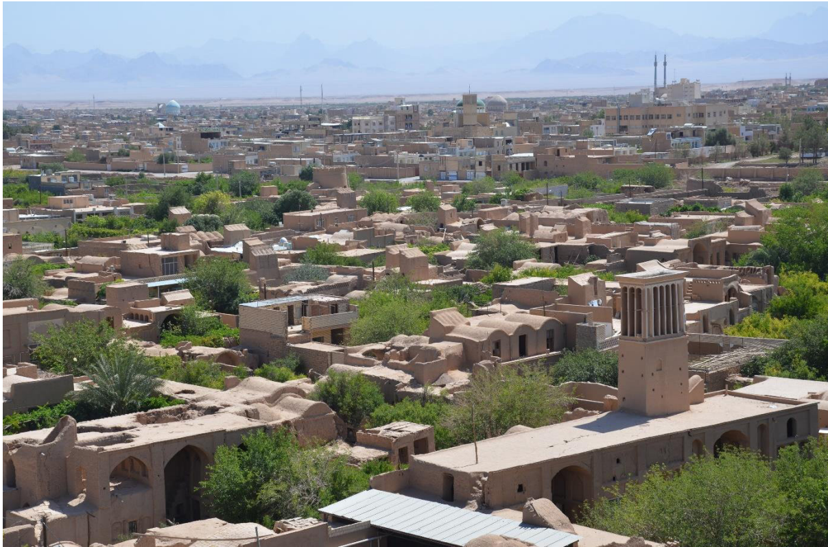
Figure 3-69: Different types of ceiling in city of Meybod. (Photo by Arsalan Chabok)
