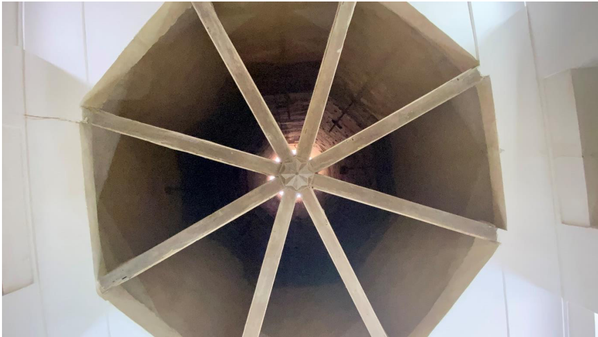
Figure 3-80: Plan of eight-sided wind catcher. (Photo by Arsalan Chabok)
