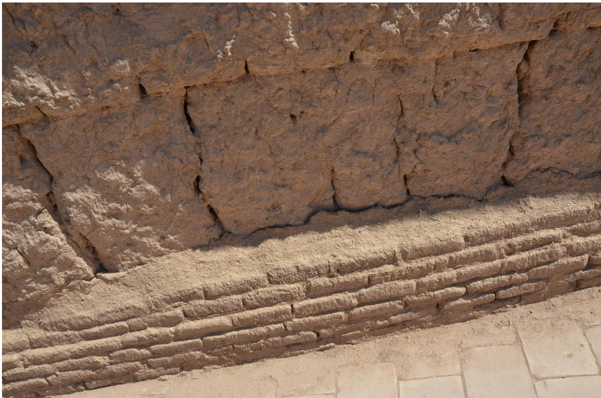
Figure 3-84: Bricks are used to build floors and walls as a base and upper level is clay. (Photo by Arsalan Chabok)
