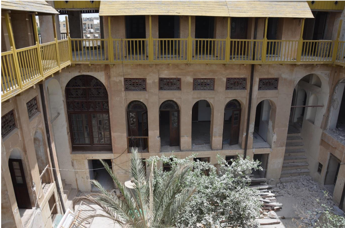
Figure 3-30: There are large openings around the central courtyard and also on the outside of this house in Bushehr. Therefore, cross Ventilation is always provided inside this building. (Photo by Arsalan Chabok)
