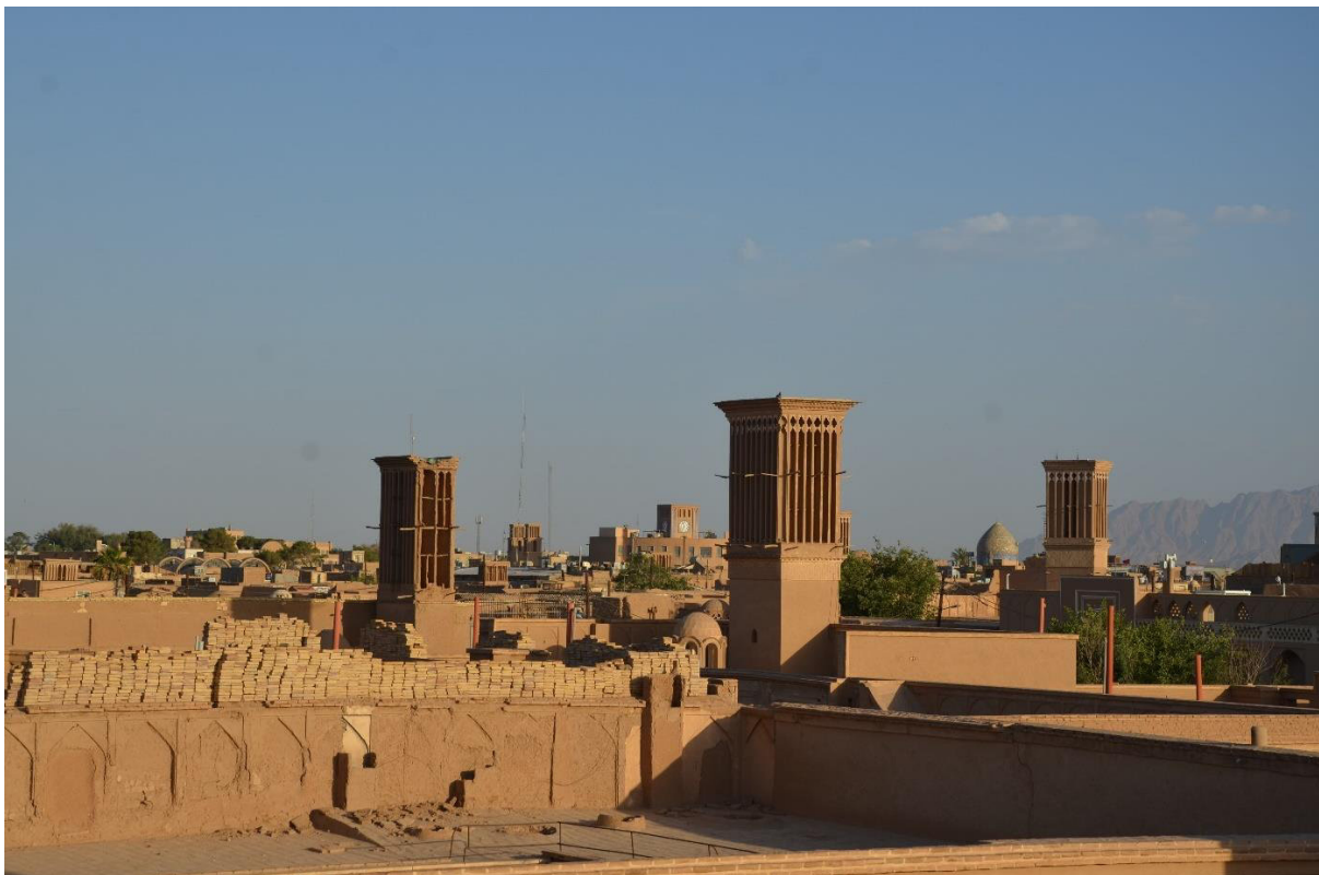
Figure 3-62: view of Yazd city with wind catchers. (Photo by Arsalan Chabok)
