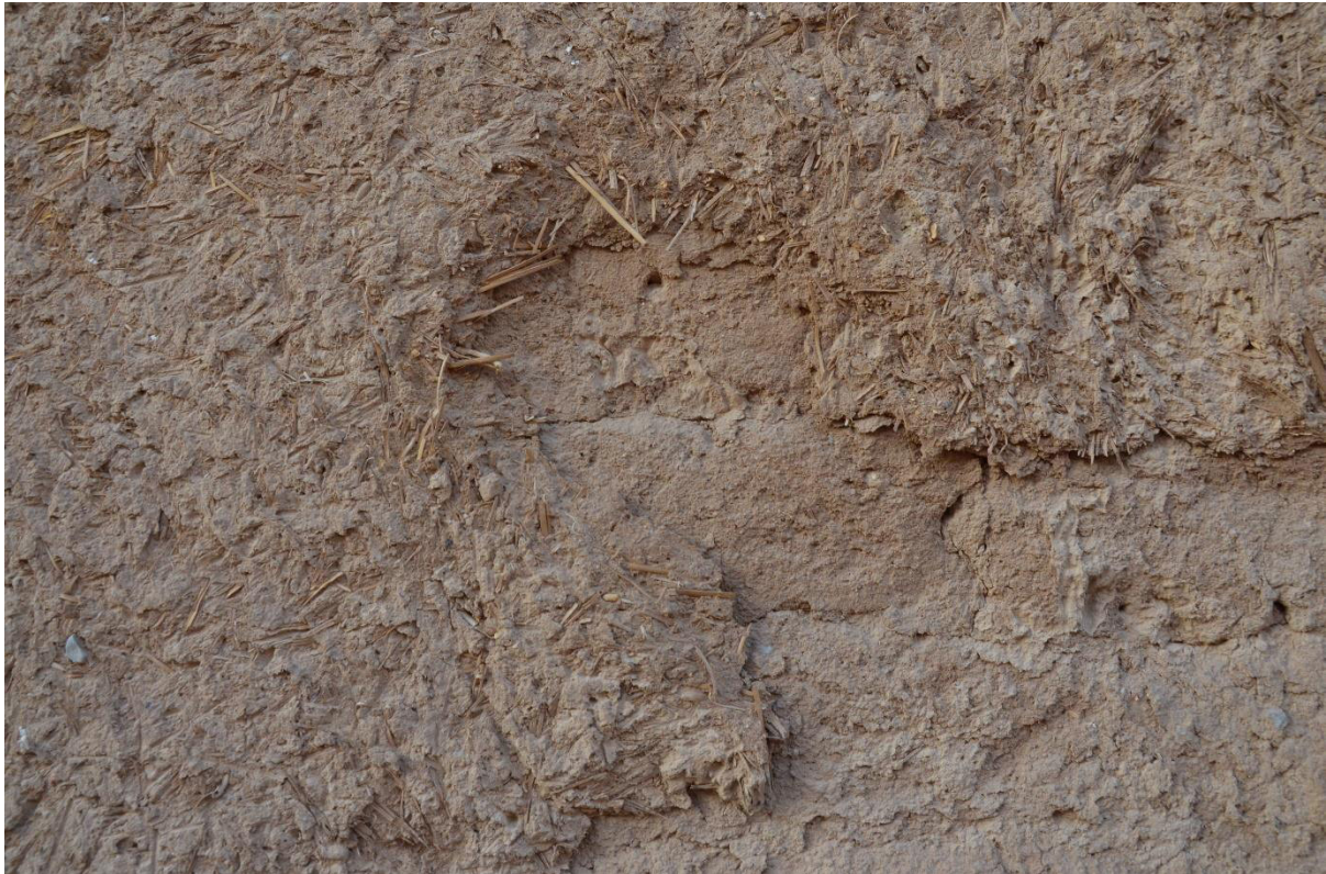
Figure 3-83: Clay is composed of dirt, water, and sometimes small particles of straw. (Photo by Arsalan Chabok)
