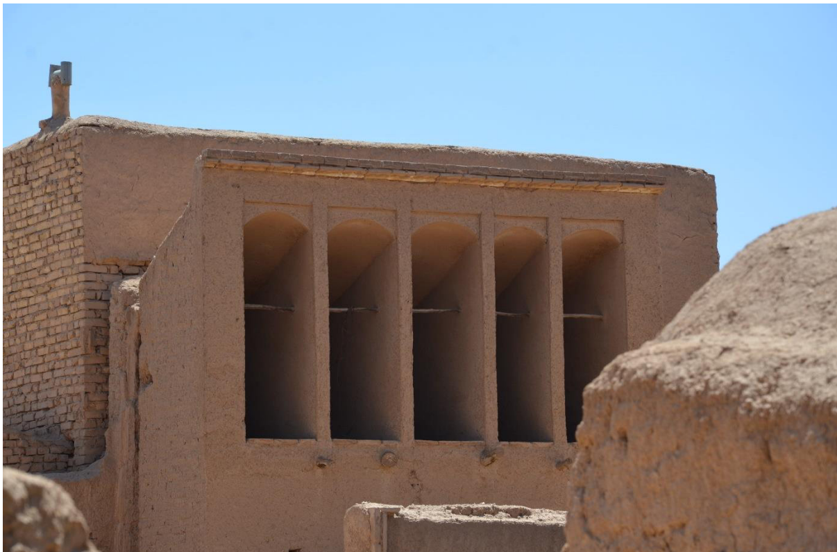
Figure 3-74: One-sided wind towers protruding from buildings in the city of Meybod near Yazd in central Iran. (Photo by Arsalan Chabok)
