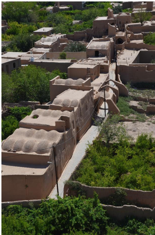
Figure 3-59: Traditional dwellings in Meybod (northern Yazd Province) are entirely enclosed from the outside. The building fabric shields the courtyard's Microclimate from the severe Macroclimate outdoors. (Photo by Arsalan Chabok)
