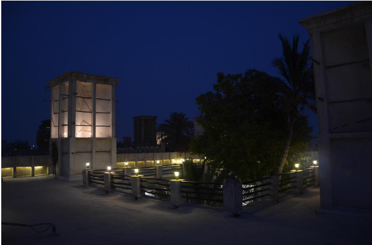
Figure 3-24: Night view of large Wind towers that receive the circulating wind between sea and land are the dominant feature of the historic port of kong in the Hormozghan Province. (Photo by Arsalan Chabok)
