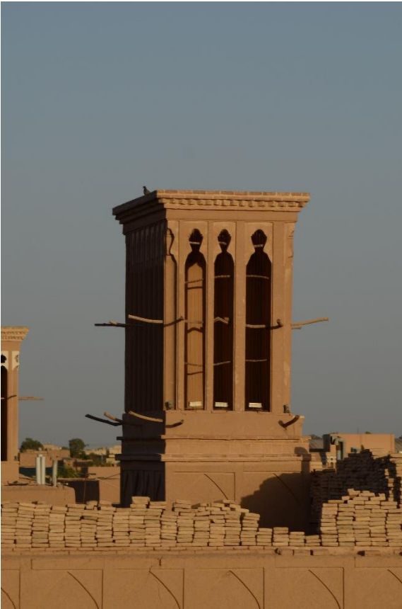
Figure 3-78: Different styles four-sided wind catcher with different ages. (Photo by Arsalan Chabok)
