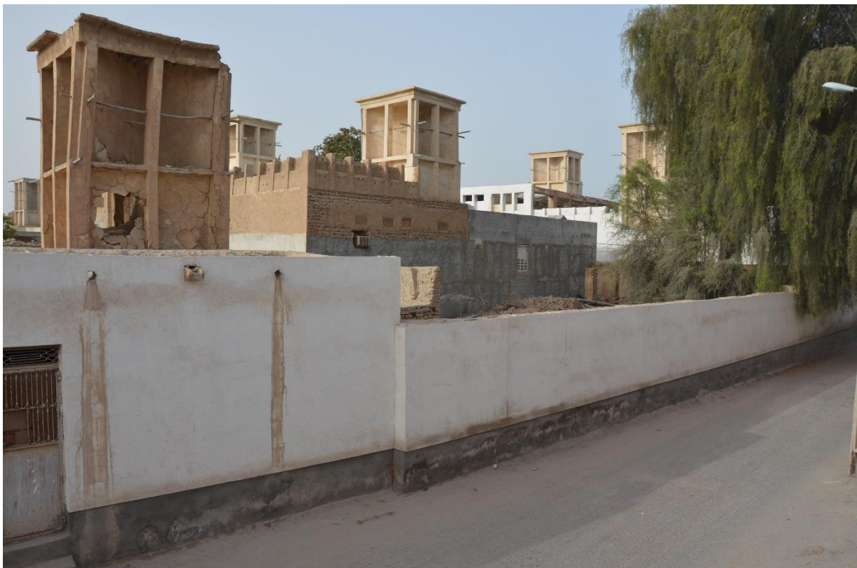
Figure 3-25: Wind towers with different materials in Kong. (Photo by Arsalan Chabok)
