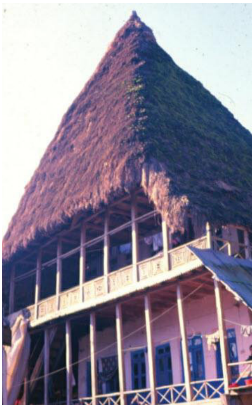
Figure 3-11: A Four-sided pyramid-shaped gable roof of a house near Langarud, in the Gilan Province. Thatch Has been used for covering the roof. (Photo by Vahid Ghobadian)
