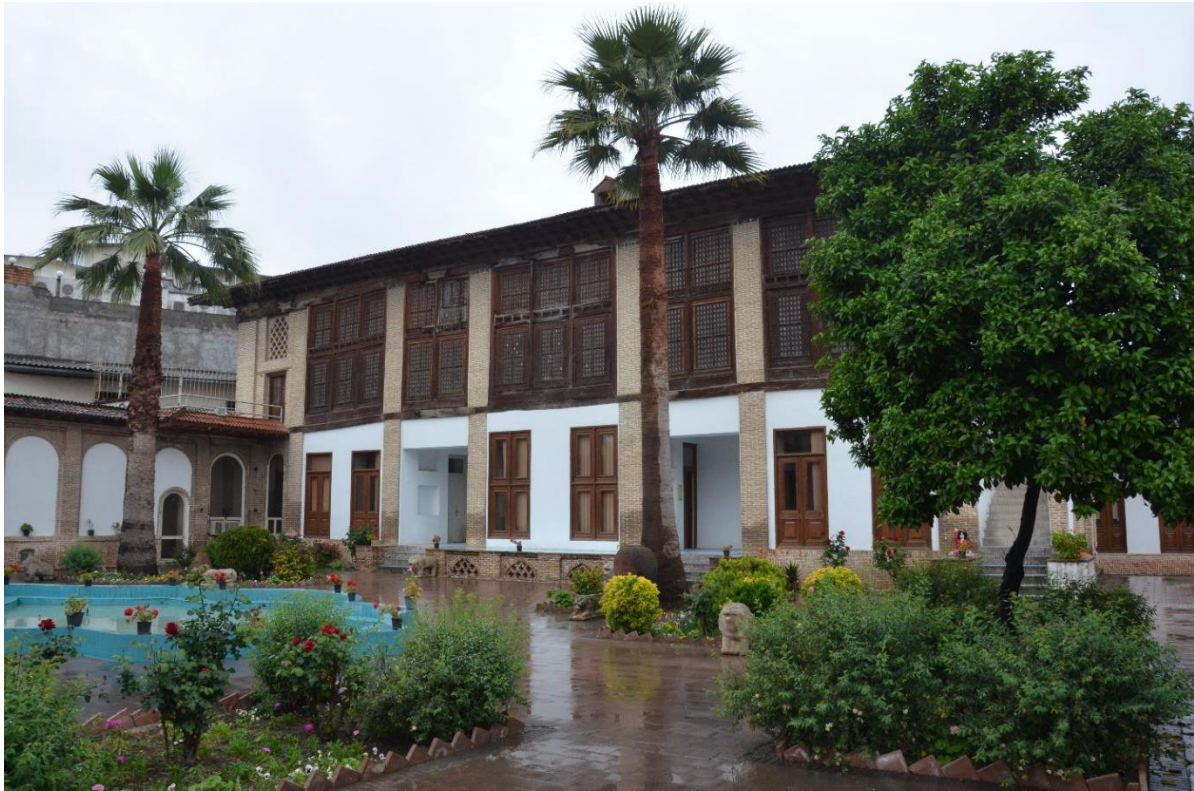
Figure 3-9: For cross ventilation, there are windows on opposite sides of all the rooms on the upper floor of the Kolbadi House in Sari. (Photo by Arsalan Chabok)
