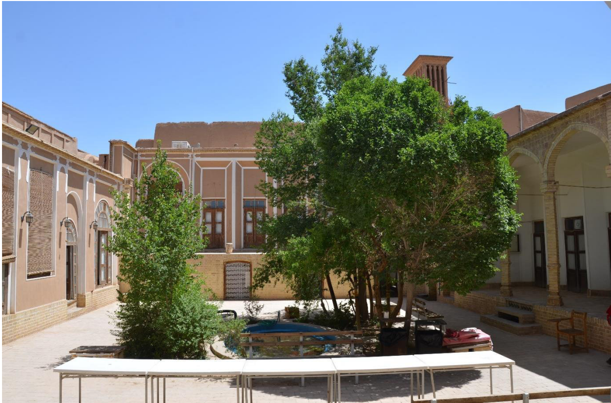
Figure 3-68: A view of the central and all the openings are open inside the courtyard. (Photo by Arsalan Chabok)
