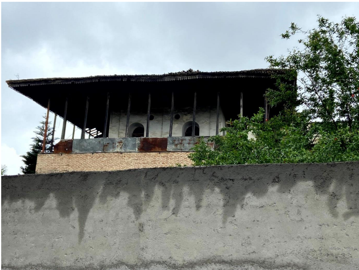
Figure 3-15: Ambulatory around the second floor in Sari, Mazandaran (Photo by Arsalan Chabok)
