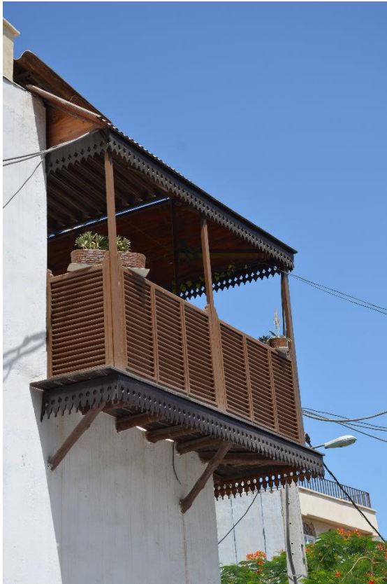
Figure 3-32: These wooden louvers, locally called Shanashil in city of Bushehr (Photo by Arsalan Chabok)
