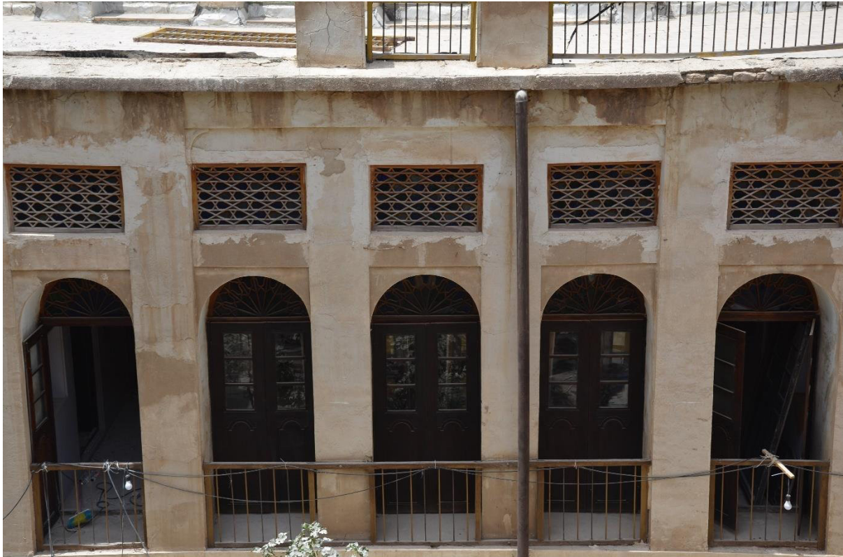
Figure 3-31: Tall opening and top of them color glass with also opening for ventilation (Photo by Arsalan Chabok)
