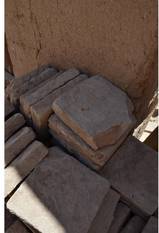
Figure 3-86: Taper wall made of clay in Meybod (Top left) use wood to keep the weight of the building (top right) not cooked brick (bottom left) cooked brick (bottom right). (Photo by Arsalan Chabok)
