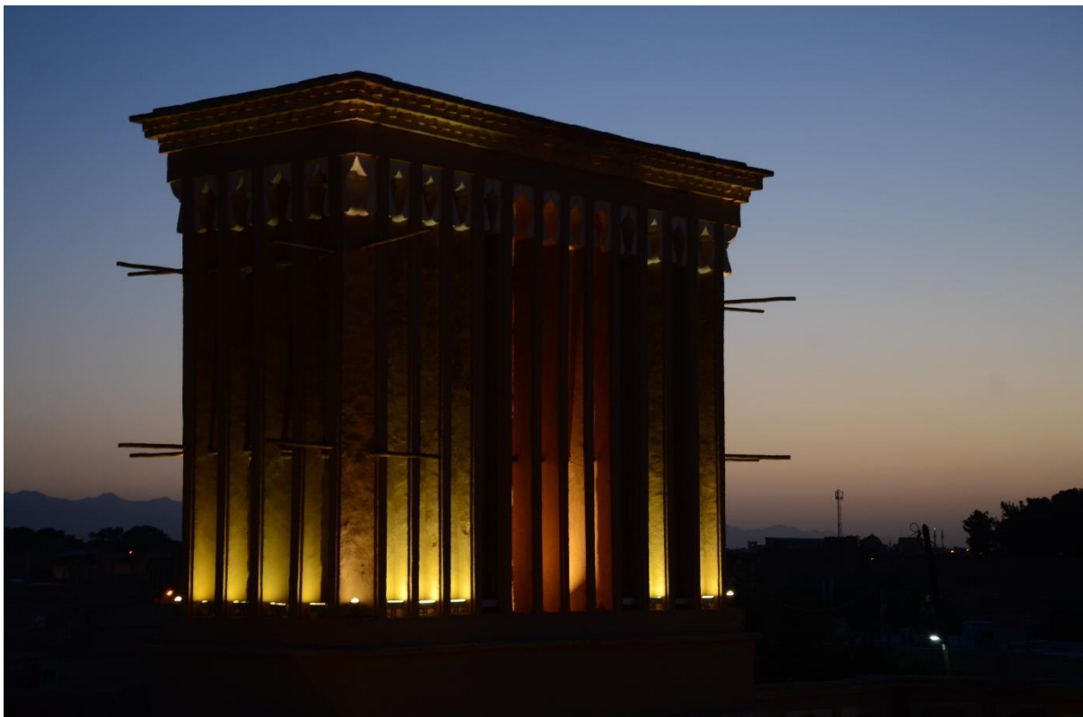
Figure 3-77: Wind catchers in night. (Photo by Arsalan Chabok)
