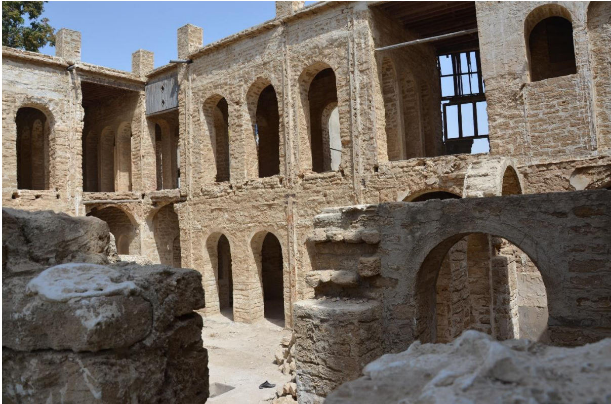
Figure 3-36: A house built with coral and sea sedimentary stones in Bushehr city. (Photo by Arsalan Chabok)
