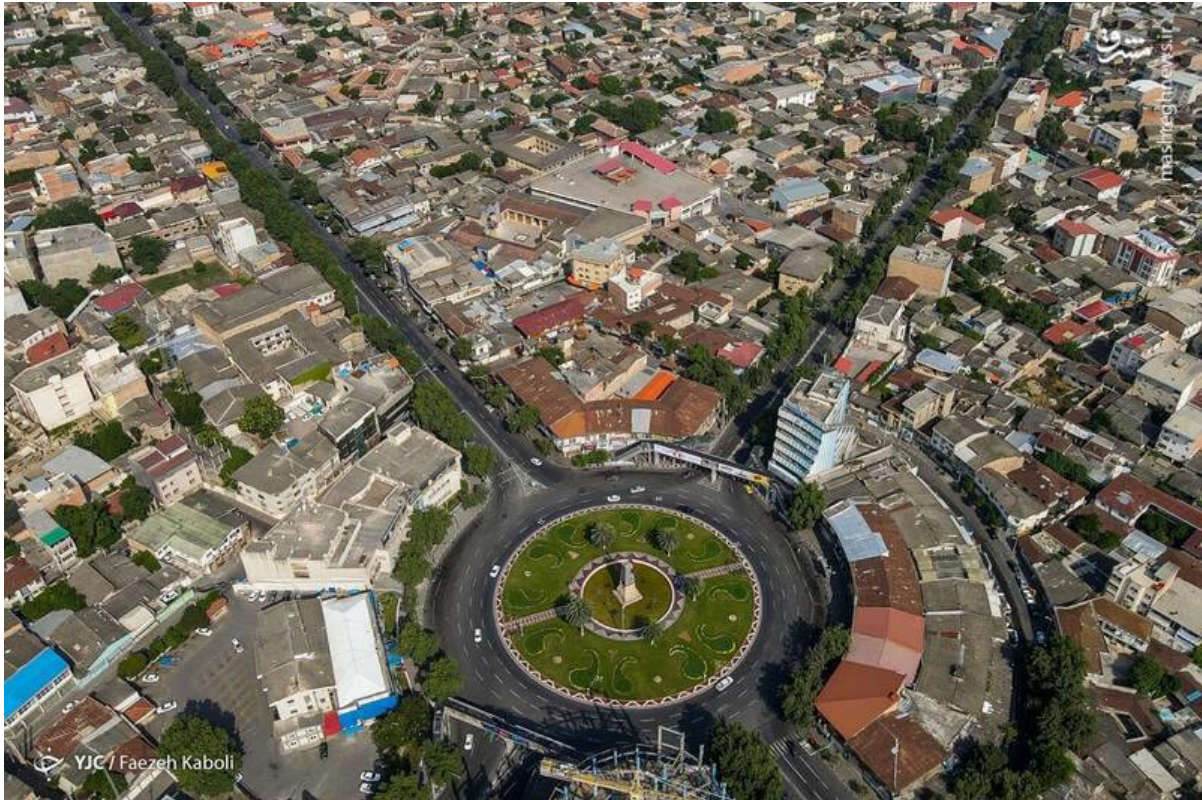
Figure 3-1: Aerial picture of the historic area of Gorgan, the provincial capital of Golestan. (Photo by Faezeh Kaboli)
