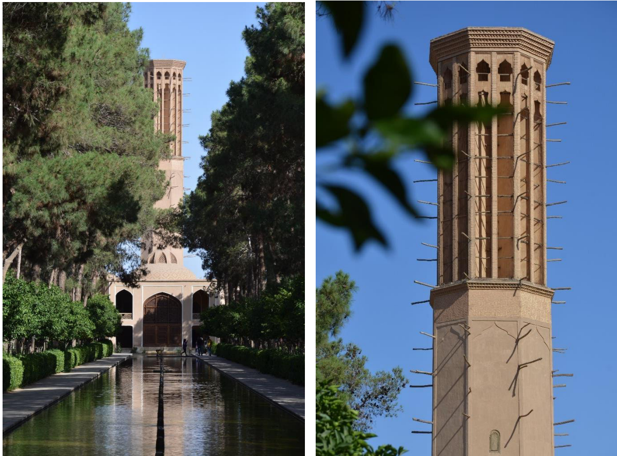
Figure 3-79: The eight-sided wind catcher of the Dolat-Abad Garden in the city of Yazd is 33 meters high, making it the tallest wind catcher in the world.
