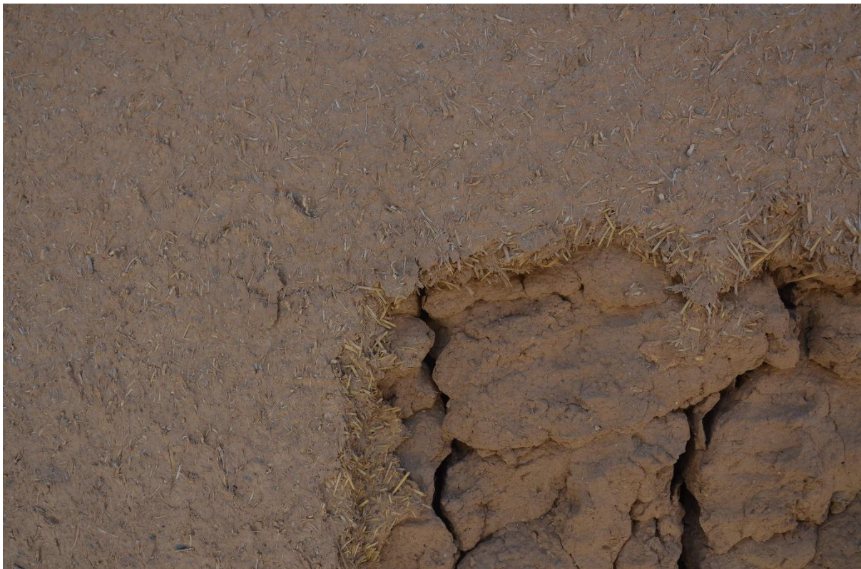
Figure 3-85: Mud wall which cover the clay. (Photo by Arsalan Chabok)
