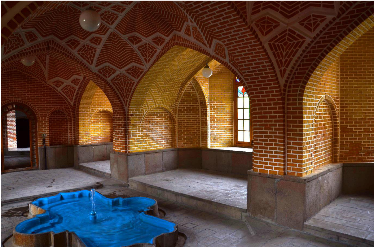
Figure 3-42: There was usually a basement below the northern side. Because of the coolness of basements in the summer, they were used especially during the summer afternoons (Photo by Arsalan Chabok)
