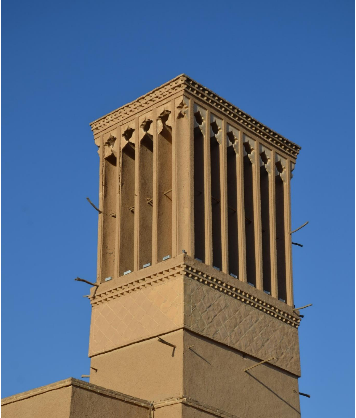
Figure 3-75: Four-sided wind tower takes in wind from one side and let air out form the other side. (Photo by Arsalan Chabok)
