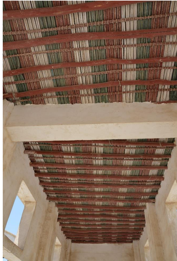
Figure 3-37: The ceiling of a residence in Bandar-e-Kong and Bushehr city is built of palm fronds joined together with ropes. On top of it is a 30centimeter layer of dirt and straw. (Photo by Arsalan Chabok)
