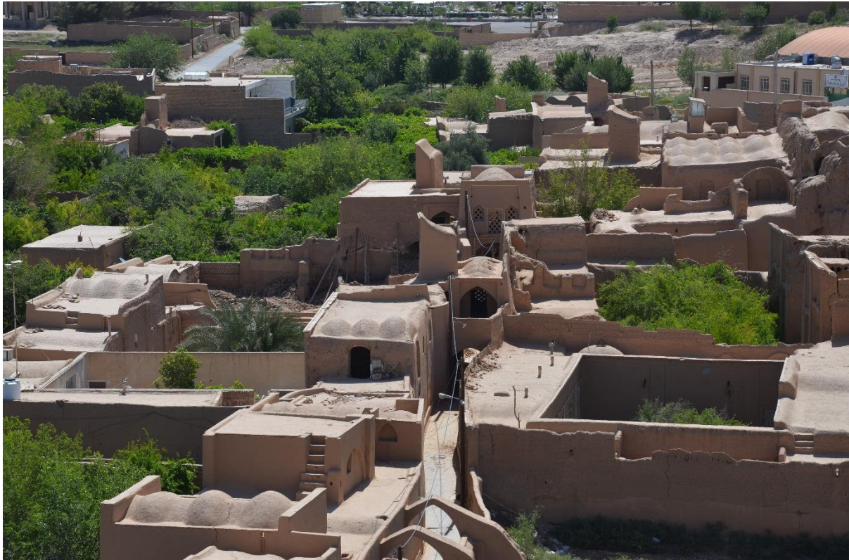
Figure 3-70: Dom style of ceilings and one-side open windcatcher in Meybod. (Photo by Arsalan Chabok)
