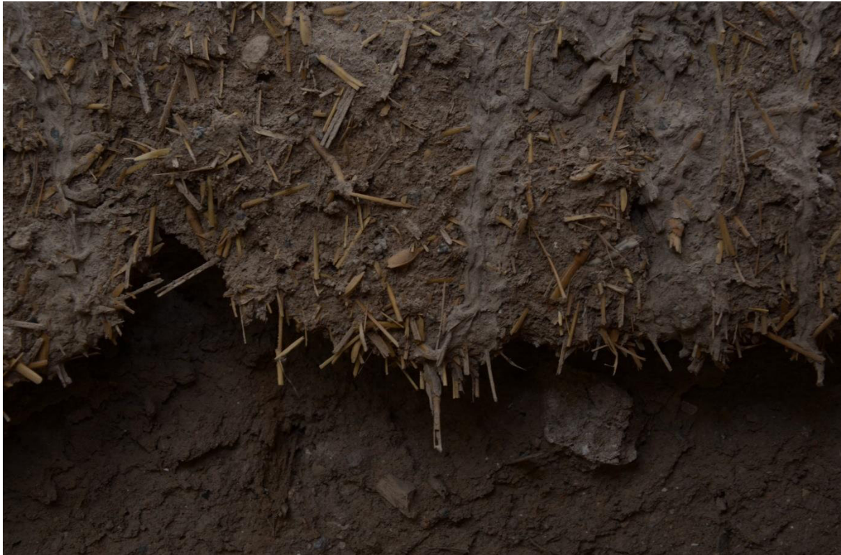
Figure 3-48: The walls were made of clay. (Photo by Arsalan Chabok)
