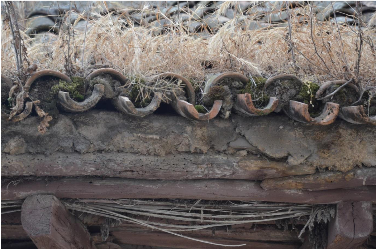
Figure 3-13: Sloping roof with cover Gali and Pottery (Photo by Arsalan Chabok)
