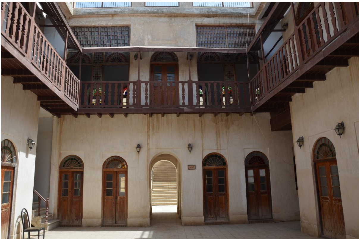
Figure 3-26: In order to shade and ventilate inside old houses in Bushehr there were long balconies and high windows all around the courtyards. (Photo by Arsalan Chabok)
