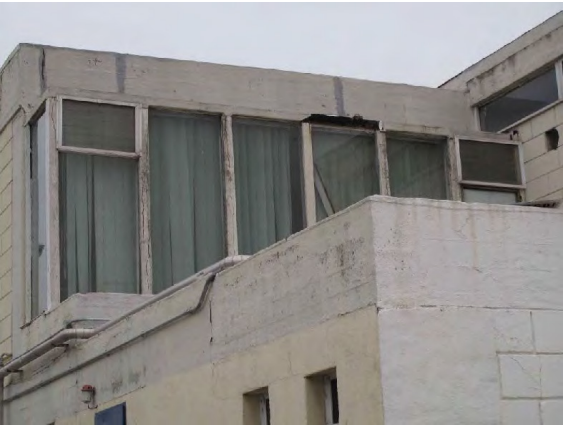
1. Very old and oxidised carpentry, which in turn produces stains on facades
