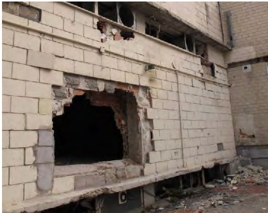
2. Holes due to the passage and anchoring of old installations
