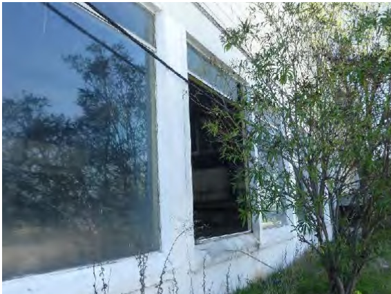
1. Broken elements and rusted carpentry appear on the glass facade
