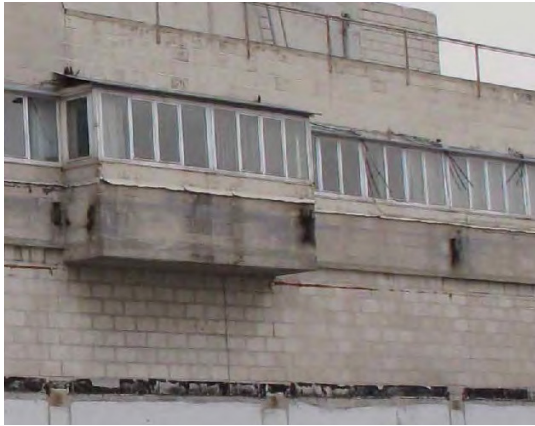
2. Serious damage due to anchoring of old structures
