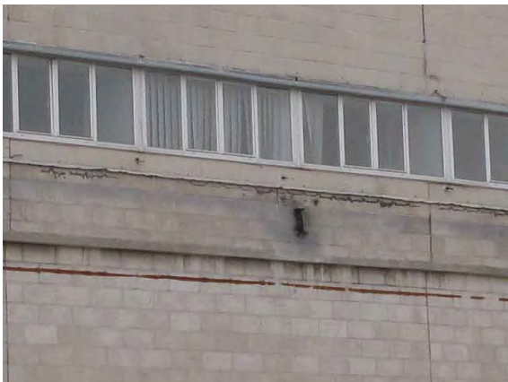
4. Damage due to anchorage of auxiliary structures
