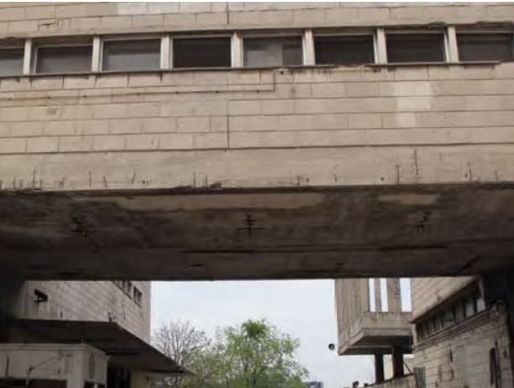
1. The bridge structure is severely damaged along its entire length, without a rusty skin reinforcement cover
