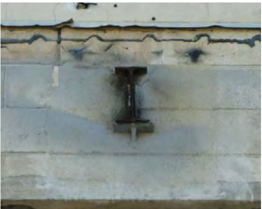
6. Damage due to anchorage of auxiliary structures
