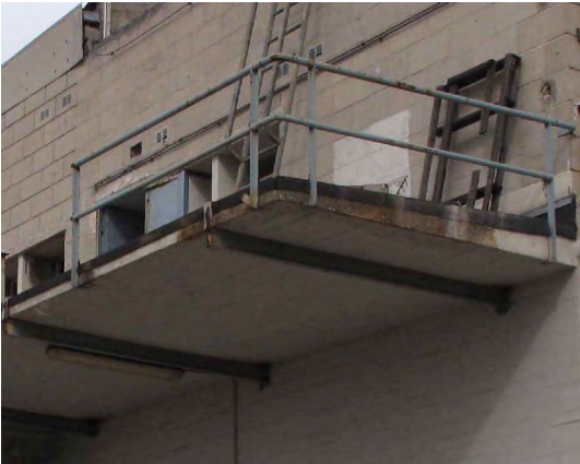
3. The metal structure of cantilever roofs shows signs of oxidation
