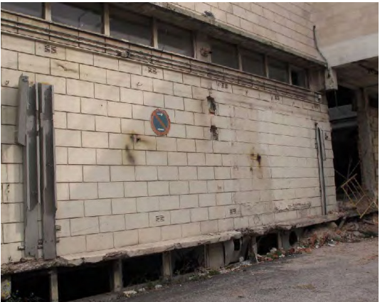
3. Decay due to anchoring of old installations
