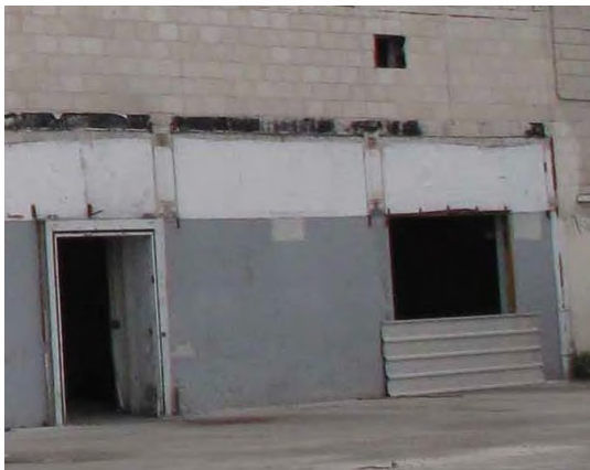
5. Absence of carpentry in doors, openings due to the exit of old installations
