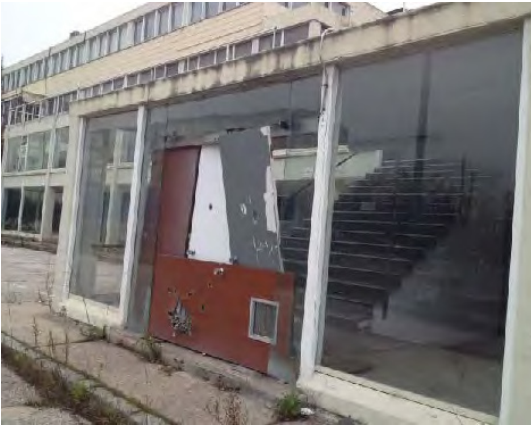
3. Absence of glass and broken pieces in the glazed walls
