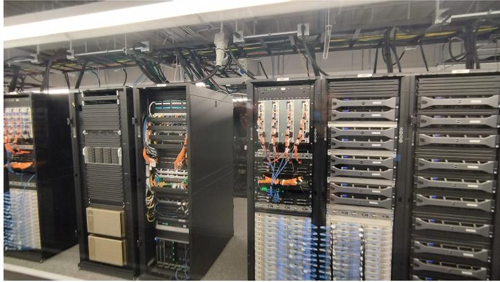
Figure 4.4: Colosseum server in the Northeastern University facilities at the Northeastern University Burlington Campus. The various sections of the structure host the SRNs, the GPUs, and the USRPs, all of them connected through the visible wires and cables.
