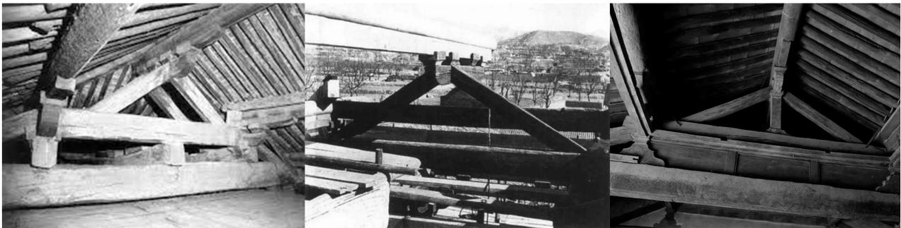
Figure 62: Left: "truss" in the Foguang temple; Middle; "truss" in the Nanchan temple; Right: "truss with *Shuzhu*" in the Longmen temple (Pan and Campbell, 2017)
