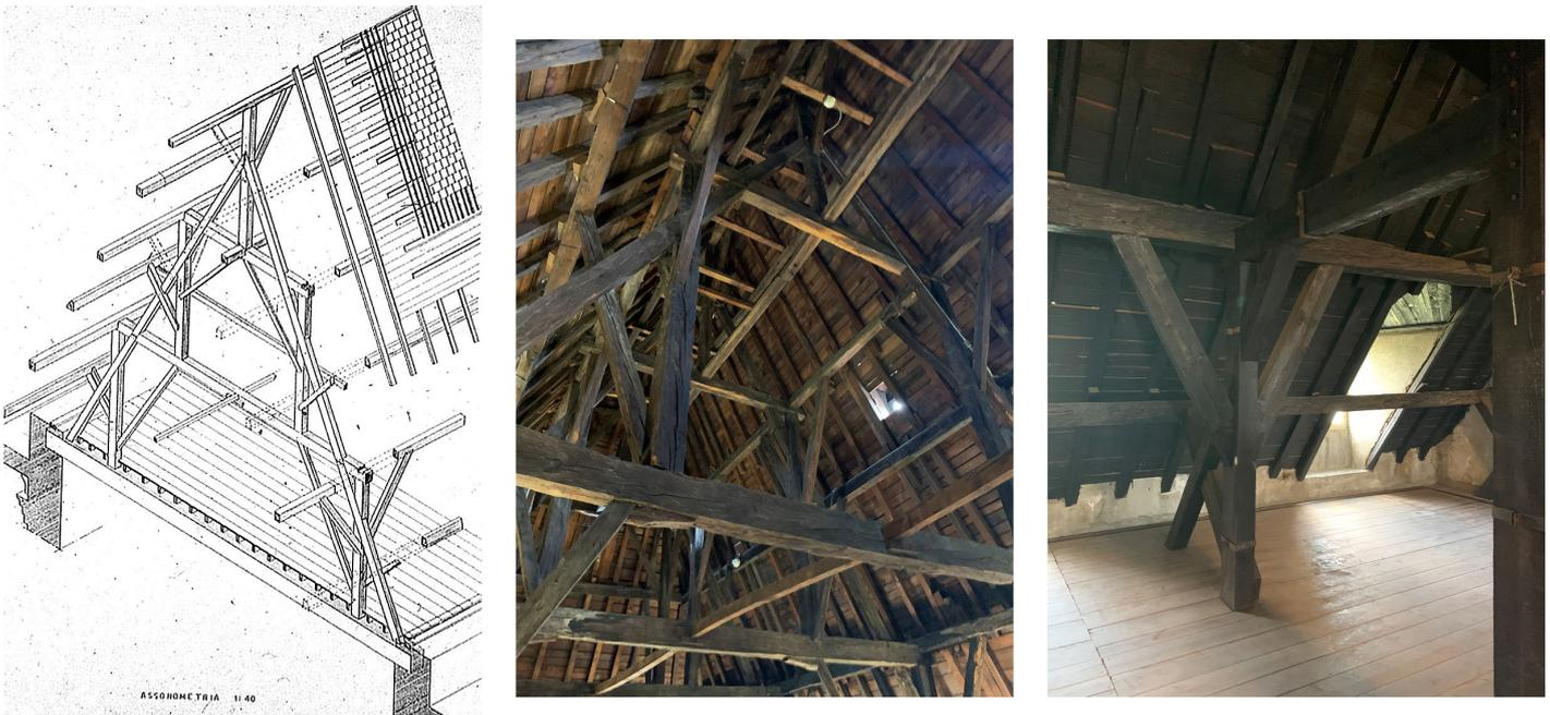
Figure 6: Left: detail of the timber frame roof of Castello di Valentino (drawing by Bertolini Cestari 1986); Right: photos of Castello di Valentino
