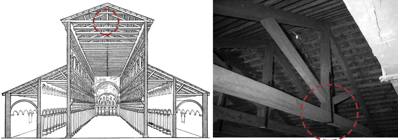
Figure 16: Left: Section of the Basilica of St. Peter (Spagnesi, 1995); Right: Detail of a closed joint truss of the Basilica St. Paul (Valeriani, 2012)
