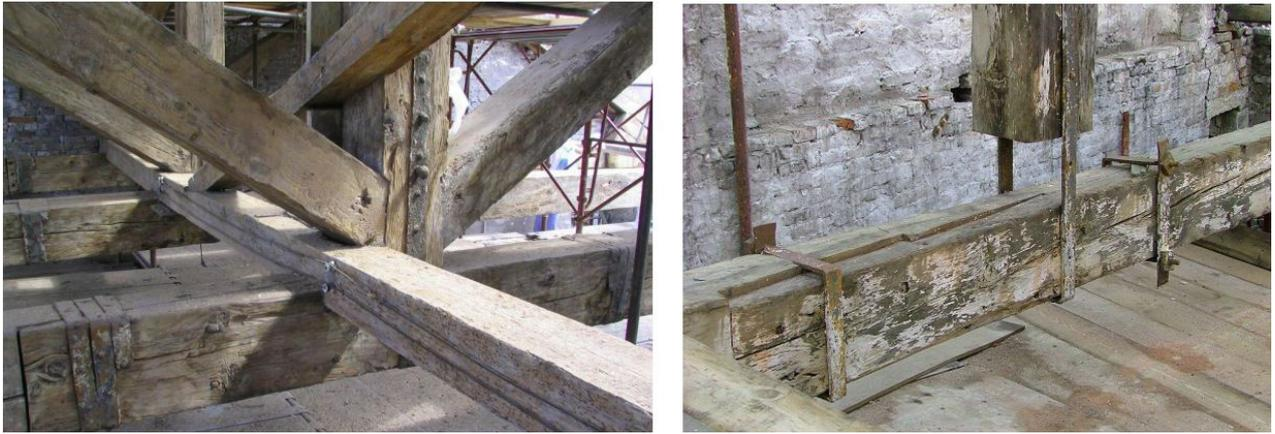
Figure 31: Survey photos (Menichelli et al, 2009) show the original connection of the post and tie beam (left) and the intervention of an open joint truss in the 19 century (right)
