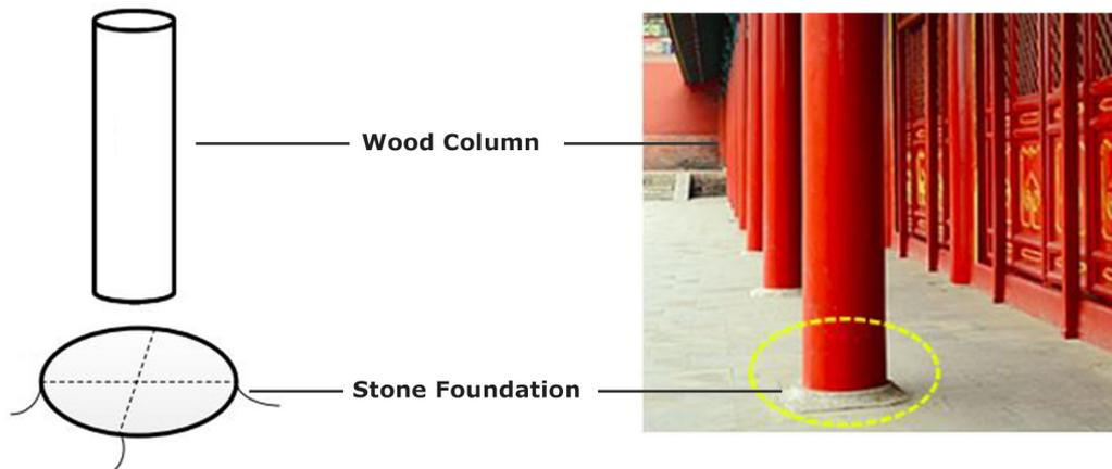
Figure 68: Wood column and stone foundation (He et al, 2017)
