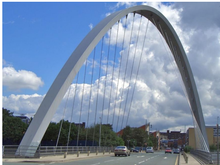
Figure 23: Hulme Arch Bridge – Manchester
