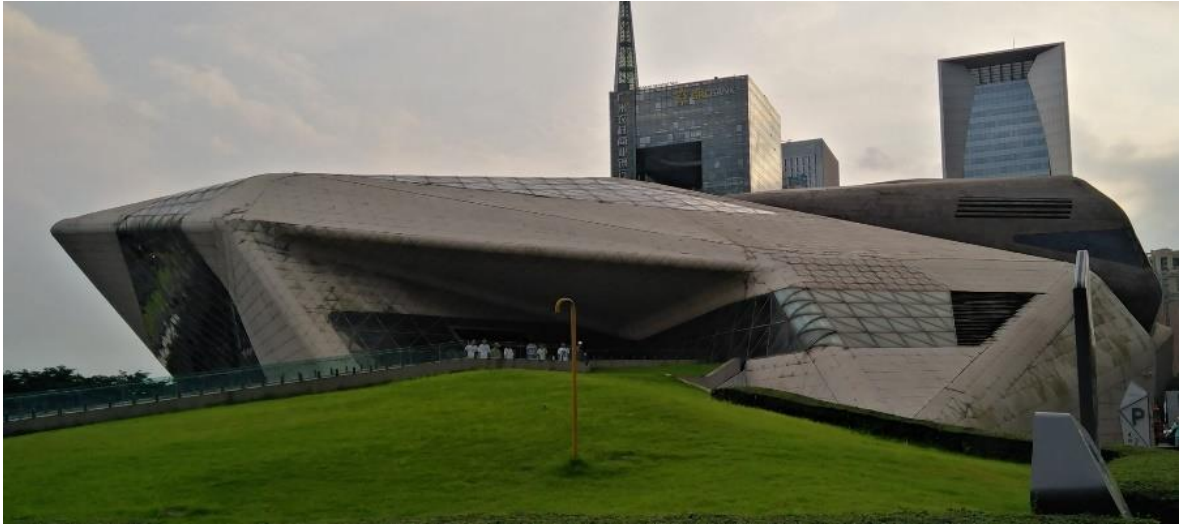
Figure 17: Guangzhou Opera House – Zaha Hadid - Cina
