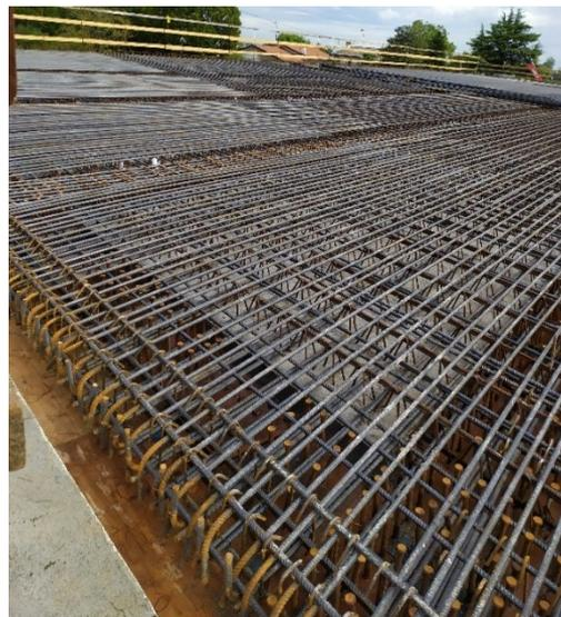
*Figure 3.4 Reinforcement displaced in the slab*
