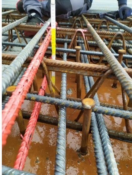
*Figure 3.6: Position of the instrumented rebar with respect to the reinforcement*
