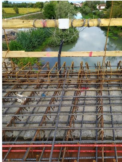
*Figure 3.7: Position of the data logger with respect to the instrumented rebars*
