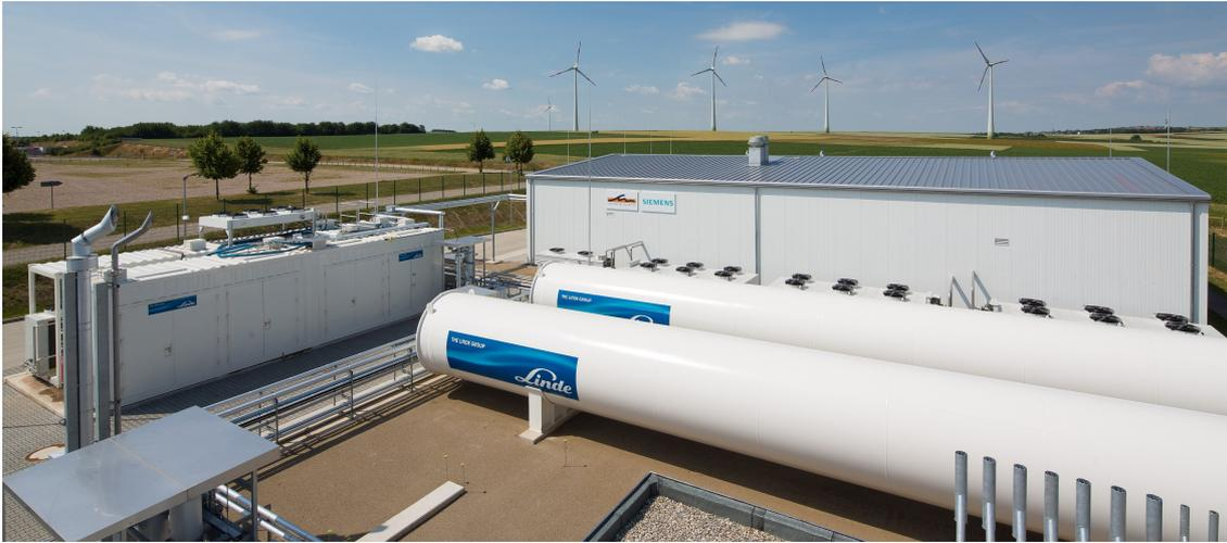
Figure 1.5. The Energiewerk Mainz - 6 MW PEMWE plant [10]
