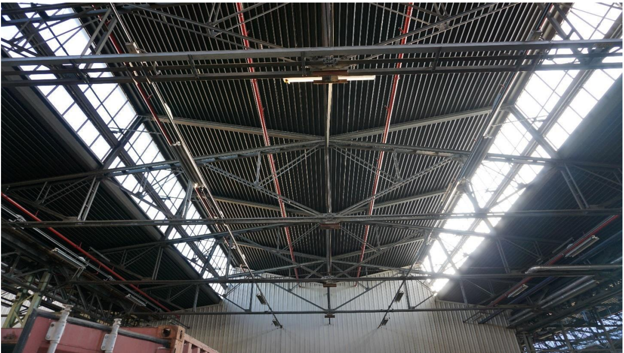
Figure 3: Internal view of the building
