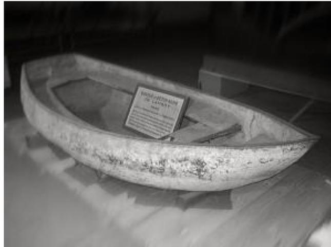
*Figura 3 - J. J. Lambot, barca in cemento armato*
