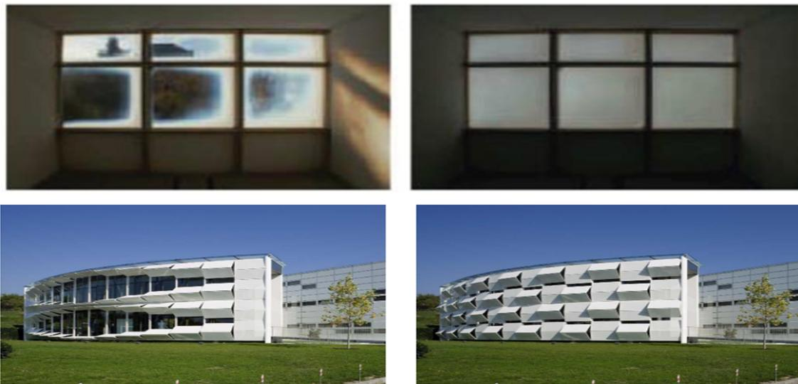
*Figure 2: Examples of adaptive and responsive envelope technologies: Thermo-tropic glazing (up) and movable solar shading (down) [8]. The movable solar shading is from Kiefertechnik Building, Ernst Giselbrecht + Partner, Styria, Austria, 2007.*
