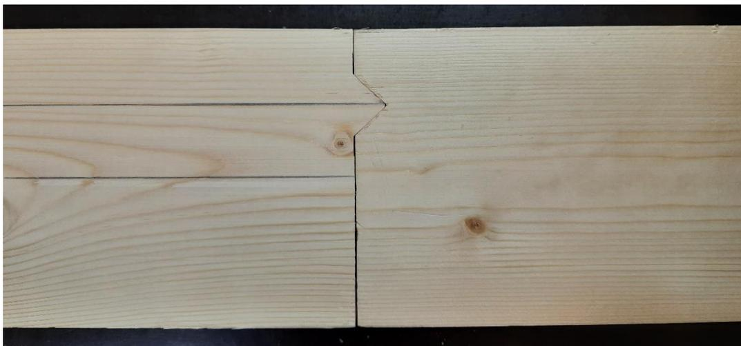
*Fig. A3: Mortise-tenon triangular shape interlocking pattern.*
