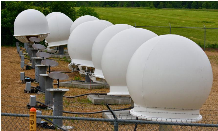
**Figure 2.12:** An array of user terminals (bottom left) and ground stations (right) that SpaceX may be using to test Starlink.
