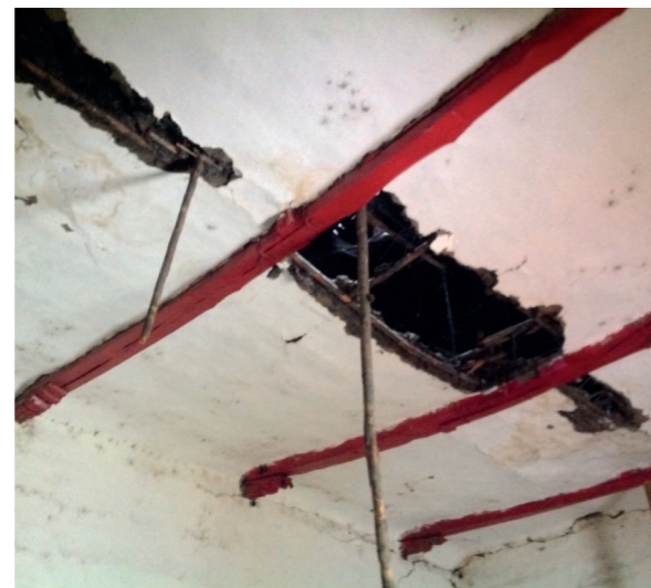
[Figure 46] Affectations due to dampness in the south wall of the presbytery (left), in the chapel, and the ceilings above the main hall, in the family house (right). Photos by CITCE, 2018.
