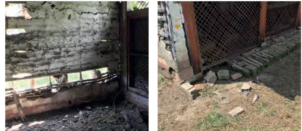
[Figure 47] Missing earth filling and disintegration of plasters of bahareque walls (left), and missing elements of the paver flooring outside the warehouse (right).
