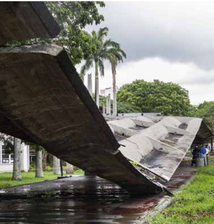
Fig. 36 Collapse of the roofed corridor. (June, 2020). Universidad Central de Venezuela (UCV). World, Cultural and Natural Heritage of Humanity by UNESCO in 2000.
