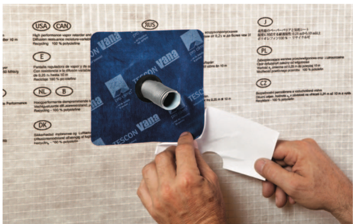
Figure 38 Airtightness layer sealing for pipes and ducts (Photo: pro clima Moll bauökologische Produkte GmbH). [5]
