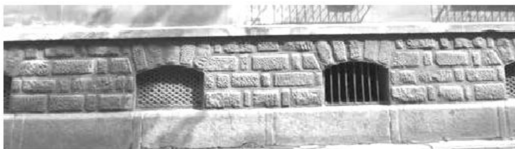
Fig.47: Dongting Street Underground Vent
