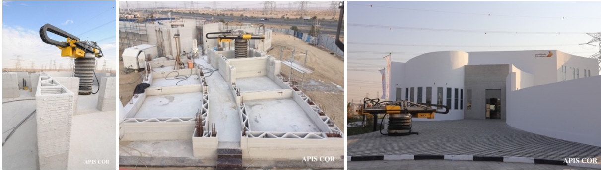
Figure 19. Construction and result of the Apis Corp Dubai project ( www.apis-cor.com/dubai-project )
