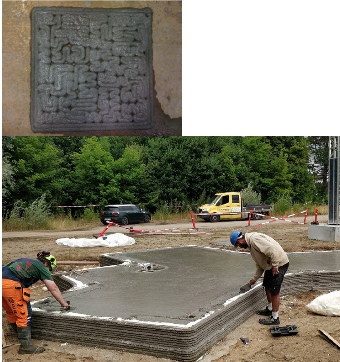
Figure 26. Example of a hatch created by an internal path on the left [51] and a perimeter filled with casted material on the right (3dcp.dk).
